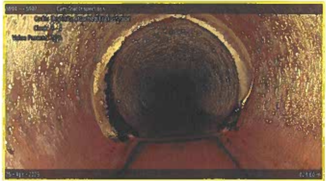
[Grade 2] Deposits Attached Encrustation at 028.60 m, 8 - 4 o'clock
