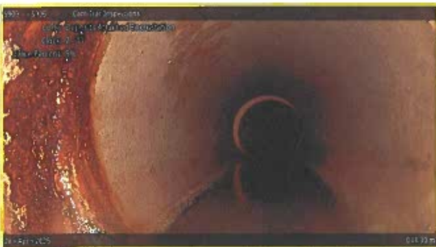
[Grade 2] Deposits Attached Encrustation at 043.30 m, 7 - 11 o'clock
