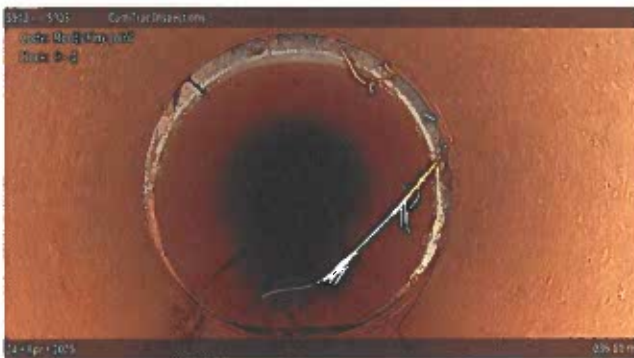
[Grade 1] Roots Fine Joint at 036.80 m, 9 - 4 o'clock
