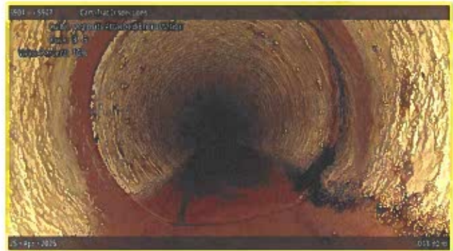
[Grade 2] Deposits Attached Encrustation at 043.80 m, 3 - 5 o'clock
