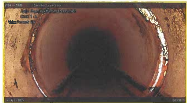
[Grade 2] Deposits Attached Encrustation at 003.90 m, 1 - 3 o'clock
