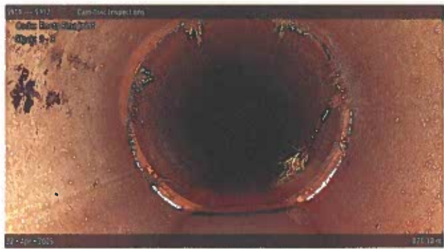
[Grade 1] Roots Fine Joint at 071.10 m, 9 - 3 o'clock
