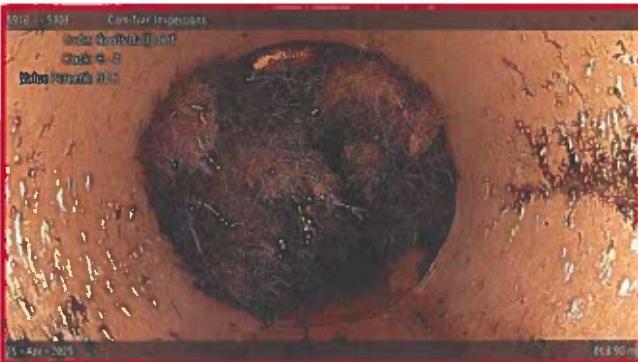
[Grade 4] Roots Ball Joint at 008.90 m, 8 - 4 o'clock
