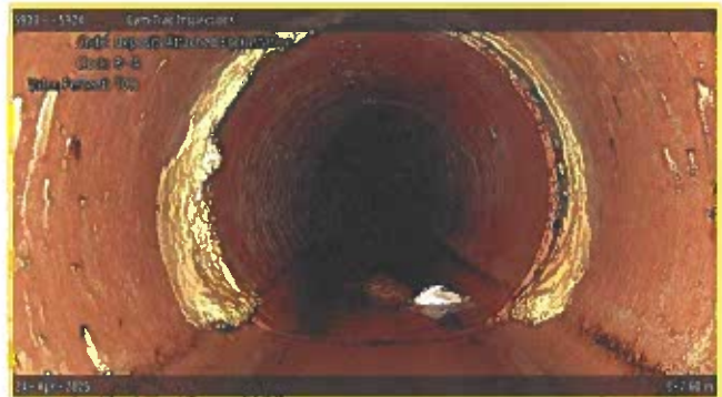
[Grade 2] Deposits Attached Encrustation at 087.60 m, 8 - 4 o'clock
