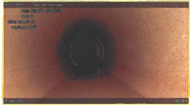
[Grade 2] Deposits Settled Fine (finish) at 024.90 m, 6 o'clock
