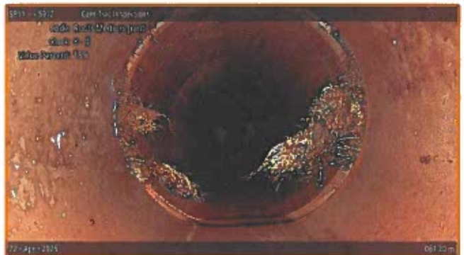
[Grade 3] Roots Medium Joint at 064.20 m, 8 - 4 o'clock
