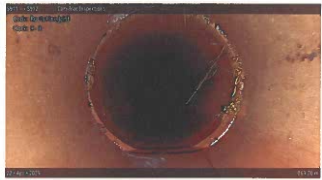
[Grade 1] Roots Fine Joint at 069.70 m, 9 - 3 o'clock
