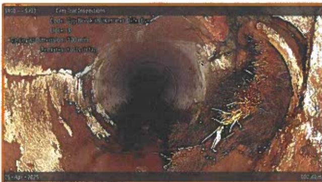
[Grade 3] Tap Break-in/Hammer Defective at 002.80 m, 3 o'clock | roots in tap
