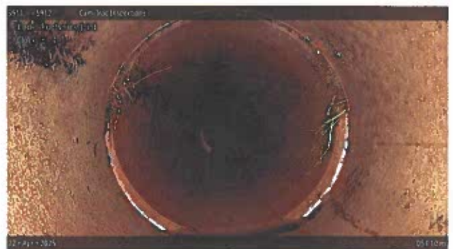
[Grade 1] Roots Fine Joint at 053.10 m, 8 - 4 o'clock
