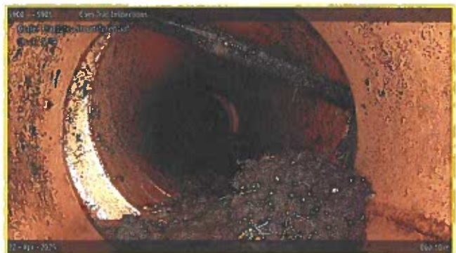
[Grade 2] Fracture Circumferential at 000.10 m, 5 - 9 o'clock
