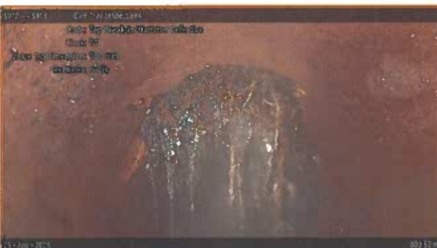
[Grade 3] Tap Break-in/Hammer Defective at 000.80 m, 11 o'clock | roots around tap
