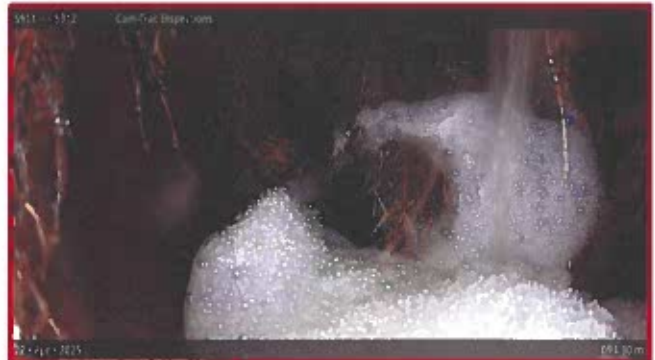
[Grade 5] Roots Ball Barrel at 094.30 m, 8 - 5 o'clock
