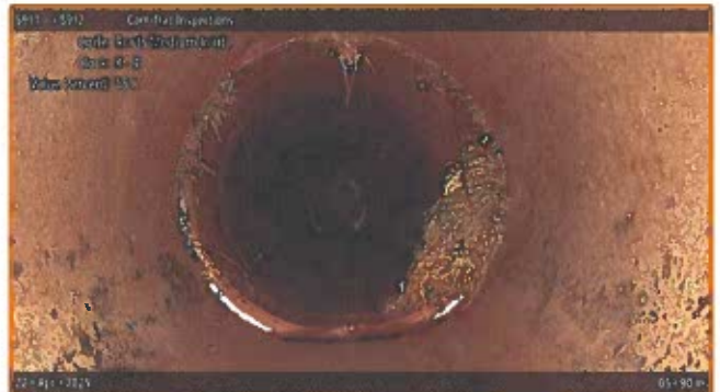
[Grade 3] Roots Medium Joint at 059.90 m, 8 - 4 o'clock
