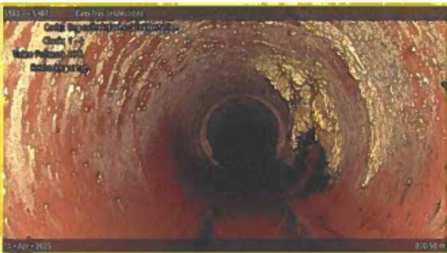
[Grade 2] Deposits Attached Encrustation at 020.50 m, 1 - 4 o'clock | at tap
