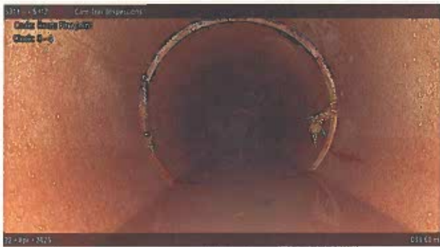
[Grade 1] Roots Fine Joint at 033.60 m, 8 - 4 o'clock
