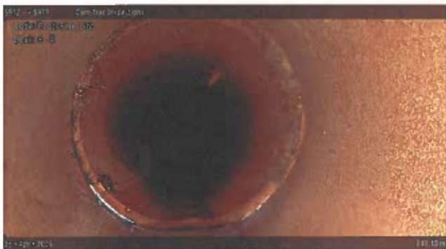
[Grade 1] Roots Fine Joint (start) at 041.40 m, 8 - 4 o'clock
