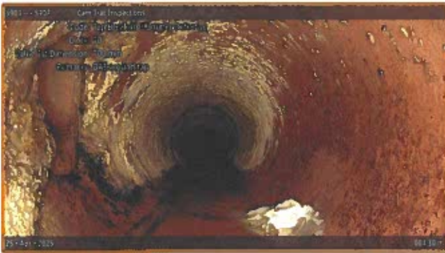
[Grade 3] Tap Break-in/Hammer Defective at 004.30 m, 10 o'clock | DAE around tap
