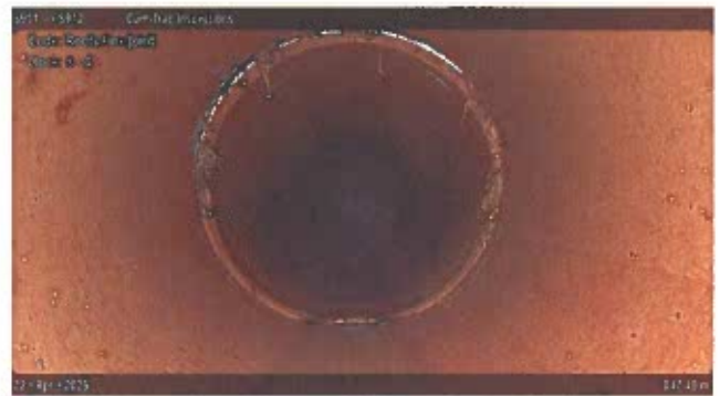
[Grade 1] Roots Fine Joint at 047.40 m, 8 - 4 o'clock
