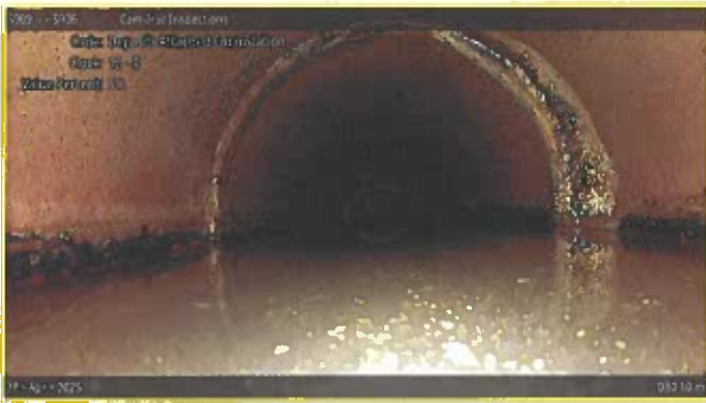
[Grade 2] Deposits Attached Encrustation at 030.10 m, 12 - 4 o'clock
