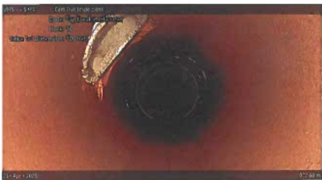
Tap Break-in/Hammer at 072.60 m, 10 o'clock
