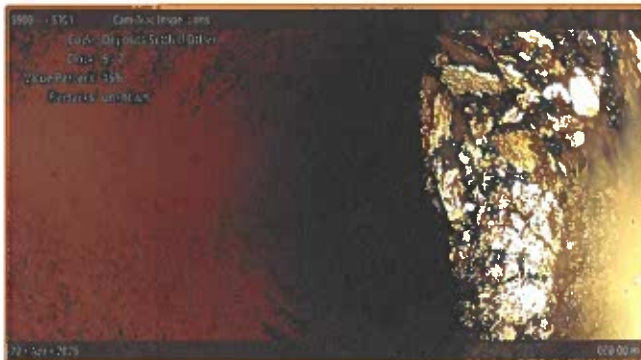
[Grade 3] Deposits Settled Other at 000.00 m, 5 - 7 o'clock | unknown
