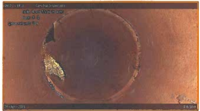
[Grade 3] Roots Medium Joint at 016.50 m, 8 - 4 o'clock
