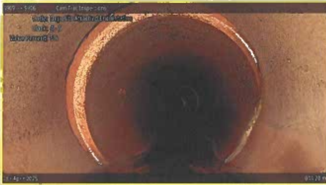
[Grade 2] Deposits Attached Encrustation at 044.20 m, 4 - 5 o'clock
