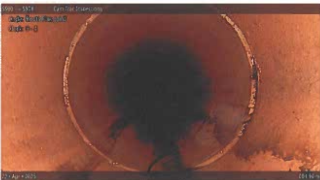
[Grade 1] Roots Fine Joint at 003.90 m, 3 - 4 o'clock
