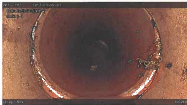
[Grade 1] Roots Fine Joint at 046.20 m, 8 - 4 o'clock
