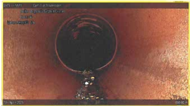
[Grade 2] Deposits Settled Gravel at 000.00 m, 6 o'clock
