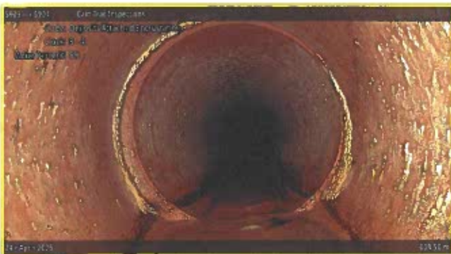
[Grade 2] Deposits Attached Encrustation at 008.50 m, 8 - 4 o'clock
