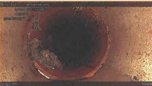
[Grade 3] Roots Medium Joint at 058.60 m, 8 - 4 o'clock
