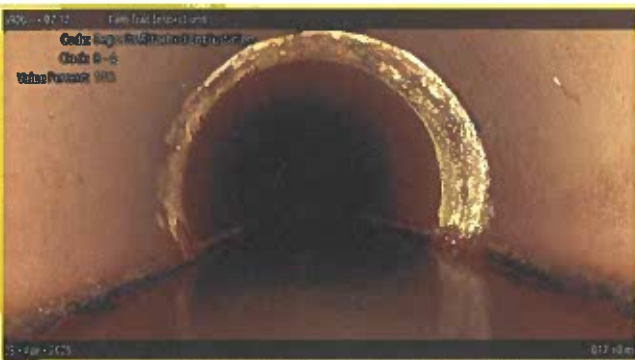
[Grade 2] Deposits Attached Encrustation at 012.80 m, 8 - 4 o'clock
