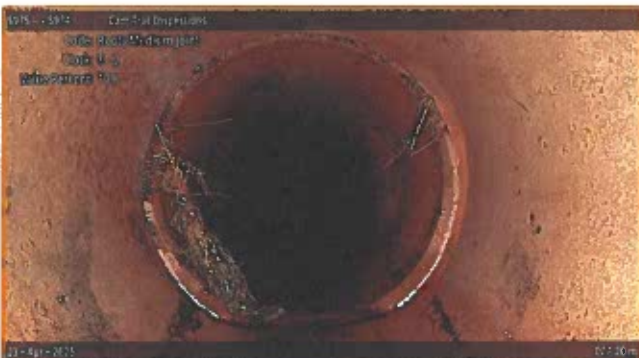
[Grade 3] Roots Medium Joint at 027.20 m, 8 - 2 o'clock
