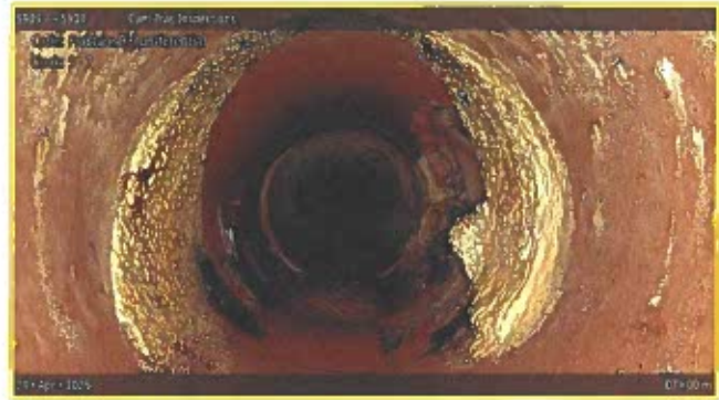
[Grade 2] Fracture Circumferential at 079.00 m, 5 - 7 o'clock
