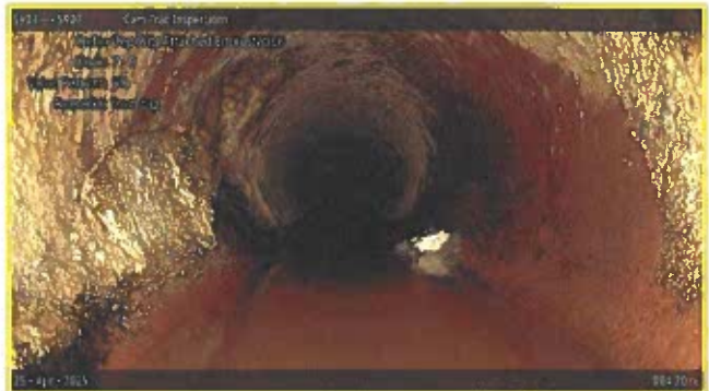
[Grade 2] Deposits Attached Encrustation at 004.20 m, 7 - 9 o'clock | around tap
