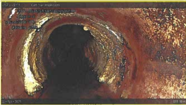
[Grade 2] Deposits Attached Encrustation at 033.30 m, 8 - 4 o'clock | at MH
