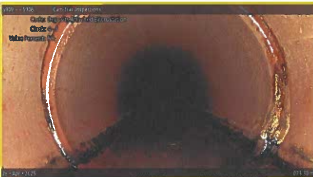
[Grade 2] Deposits Attached Encrustation at 023.30 m, 4 - 5 o'clock
