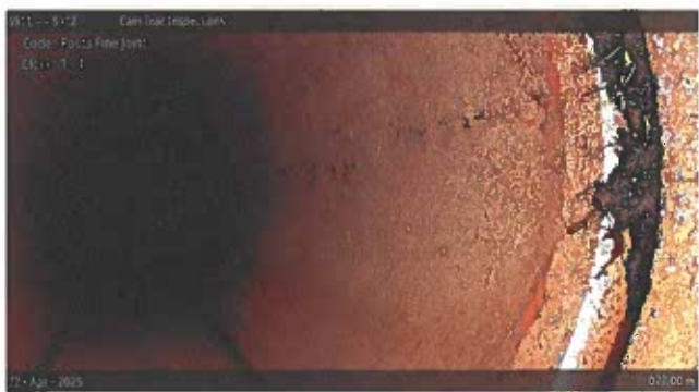
[Grade 1] Roots Fine Joint at 077.00 m, 1 - 4 o'clock
