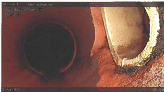
[Grade 1] Roots Fine Connection at 004.40 m, 2 - 4 o'clock
