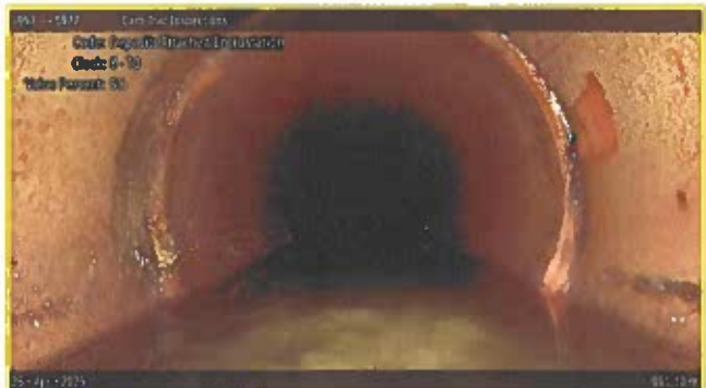
[Grade 2] Deposits Attached Encrustation at 001.10 m, 8 - 10 o'clock
