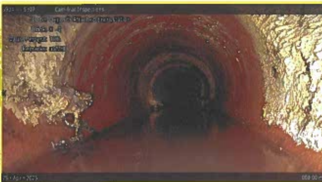
[Grade 2] Deposits Attached Encrustation at 000.00 m, 8 - 4 o'clock | at MH
