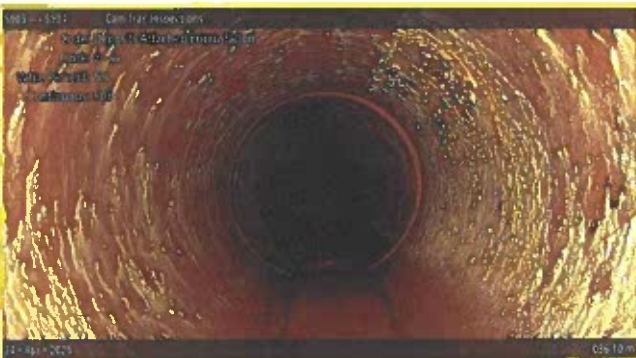
[Grade 2] Deposits Attached Encrustation (finish) at 086.10 m, 8 - 4 o'clock
