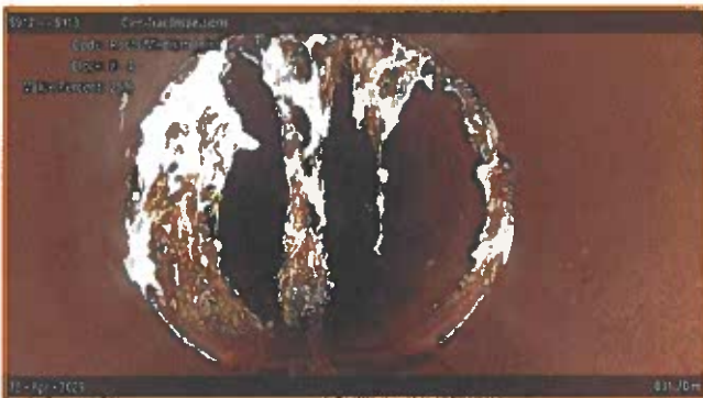
[Grade 3] Roots Medium Joint at 031.70 m, 8 - 4 o'clock
