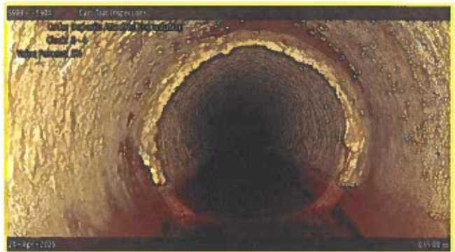
[Grade 2] Deposits Attached Encrustation at 035.00 m, 8 - 4 o'clock
