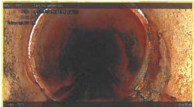
[Grade 2] Deposits Attached Encrustation at 016.20 m, 2 - 5 o'clock
