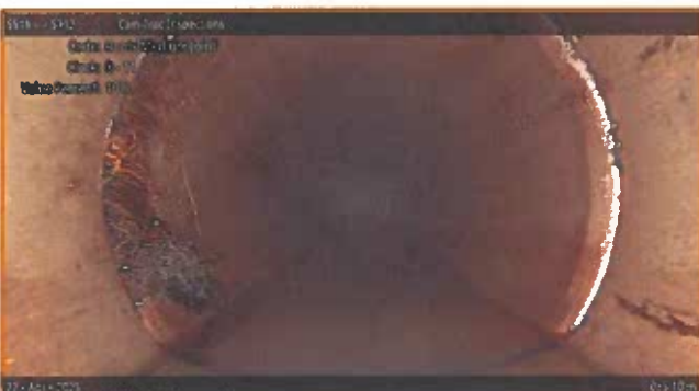
[Grade 3] Roots Medium Joint at 085.10 m, 8 - 11 o'clock
