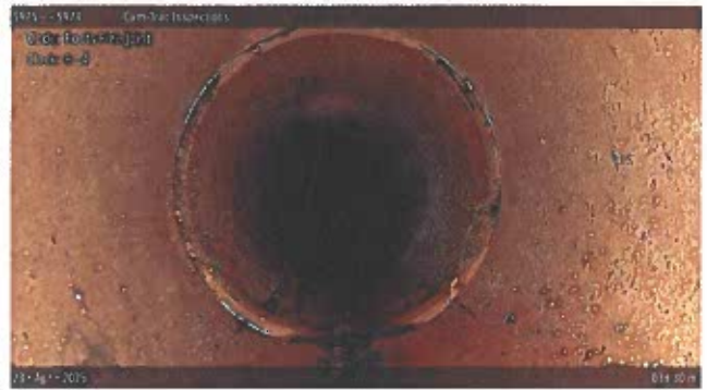
[Grade 1] Roots Fine Joint at 038.30 m, 8 - 4 o'clock
