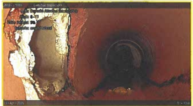
[Grade 2] Deposits Attached Encrustation at 018.40 m, 8 - 11 o'clock | around lateral
