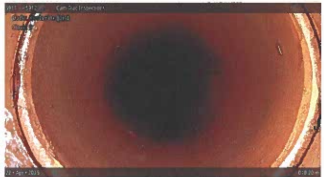
[Grade 1] Roots Fine Joint at 010.20 m, 9 o'clock
