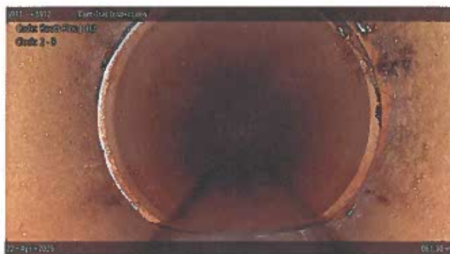
[Grade 1] Roots Fine Joint at 081.30 m, 8 - 4 o'clock
