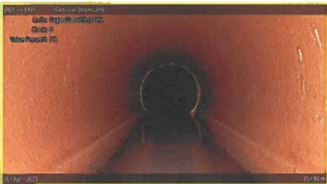
[Grade 2] Deposits Settled Fine at 059.90 m, 6 o'clock
