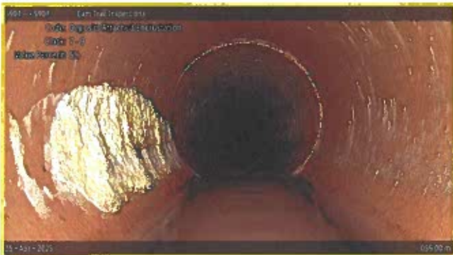
[Grade 2] Deposits Attached Encrustation at 056.00 m, 7 - 9 o'clock
