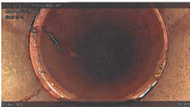
[Grade 1] Roots Fine Joint at 044.80 m, 8 - 4 o'clock
