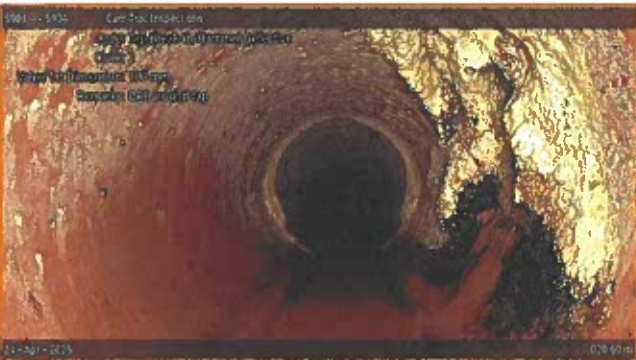
[Grade 3] Tap Break-in/Hammer Defective at 020.60 m, 2 o'clock | DAE around tap
