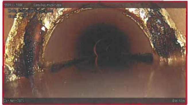
[Grade 5] Infiltration Gusher Joint at 048.40 m, 8 - 10 o'clock
