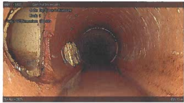
Tap Break-in/Hammer at 055.80 m, 9 o'clock
