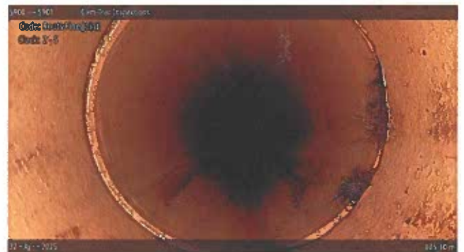
[Grade 1] Roots Fine Joint at 005.30 m, 2 - 5 o'clock
