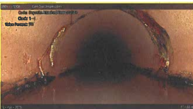
[Grade 2] Deposits Attached Encrustation at 027.60 m, 1 - 4 o'clock
