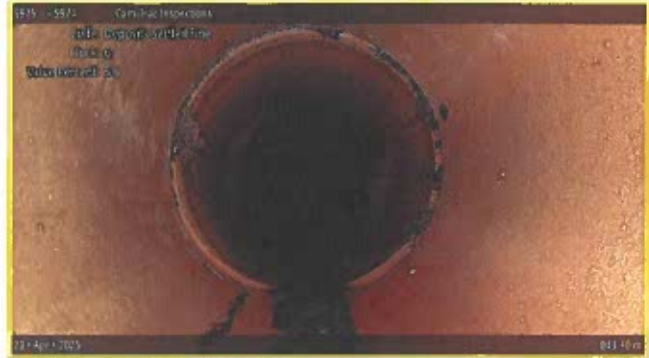
[Grade 2] Deposits Settled Fine at 043.80 m, 6 o'clock
