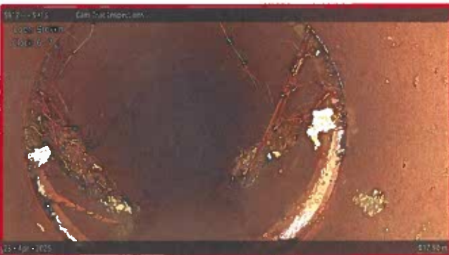
[Grade 4] Broken at 017.90 m, 6 - 7 o'clock
