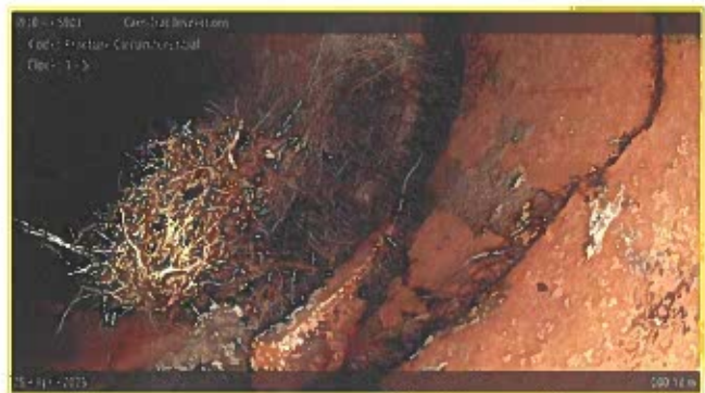
[Grade 2] Fracture Circumferential at 000.10 m, 1 - 5 o'clock
