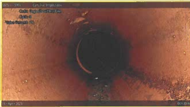
[Grade 2] Deposits Settled Fine at 003.30 m, 6 o'clock
