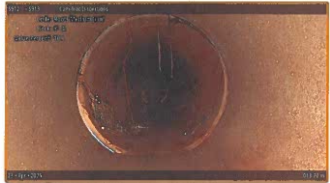
[Grade 3] Roots Medium Joint at 013.70 m, 8 - 4 o'clock
