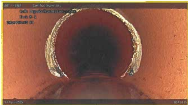
[Grade 2] Deposits Attached Encrustation at 058.90 m, 8 - 4 o'clock
