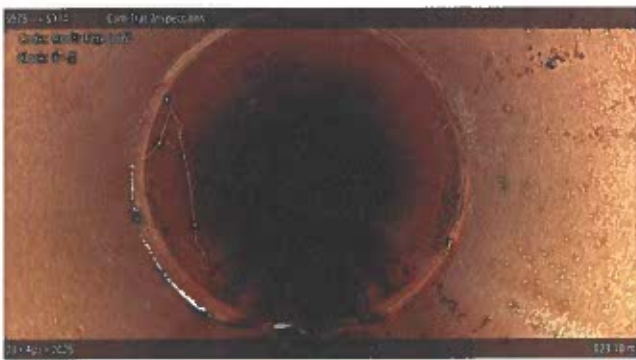
[Grade 1] Roots Fine Joint at 023.10 m, 8 - 4 o'clock
