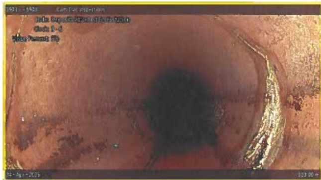
[Grade 2] Deposits Attached Encrustation at 000.00 m, 3 - 6 o'clock
