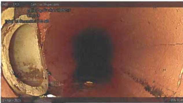
Tap Break-in/Hammer at 066.70 m, 9 o'clock
