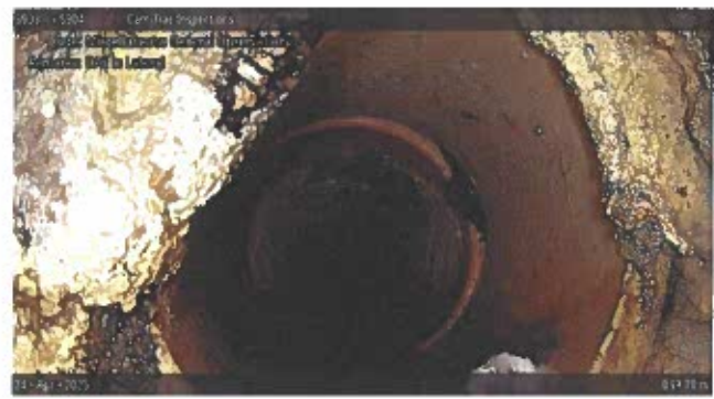
Miscellaneous General Observation at 039.70 m | DAE in Lateral
