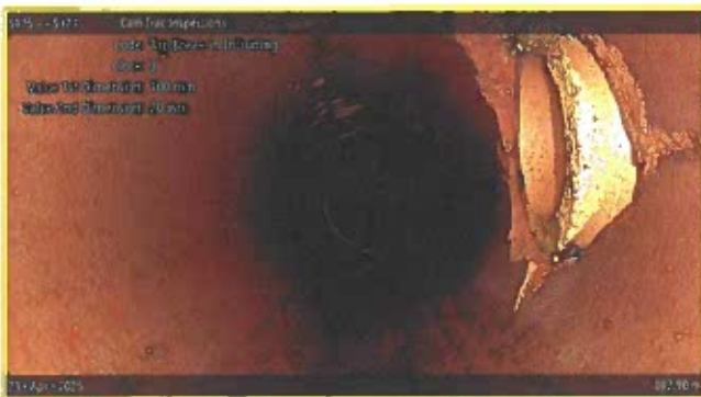
[Grade 2] Tap Break-in Intruding at 002.90 m, 3 o'clock
