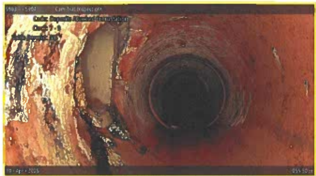
[Grade 2] Deposits Attached Encrustation at 055.50 m, 7 - 9 o'clock
