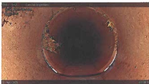
[Grade 1] Roots Fine Joint at 080.00 m, 8 - 3 o'clock
