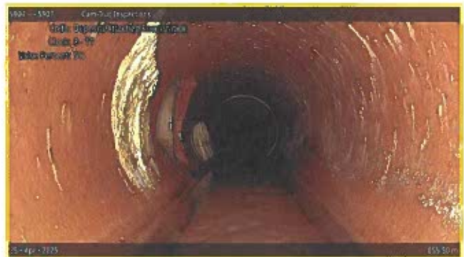
[Grade 2] Deposits Attached Encrustation at 055.50 m, 8 - 11 o'clock
