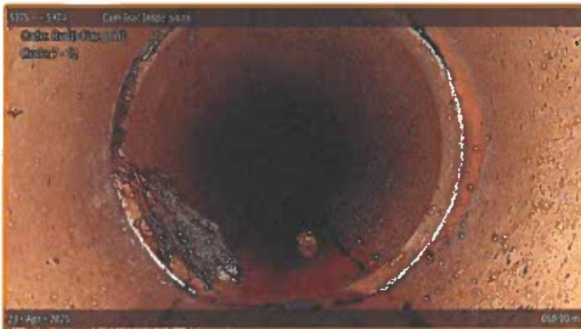
[Grade 3] Roots Medium Joint at 050.90 m, 7 - 12 o'clock
