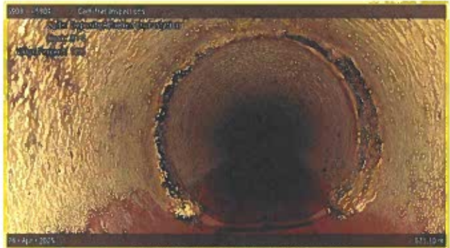
[Grade 2] Deposits Attached Encrustation at 071.10 m, 8 - 4 o'clock
