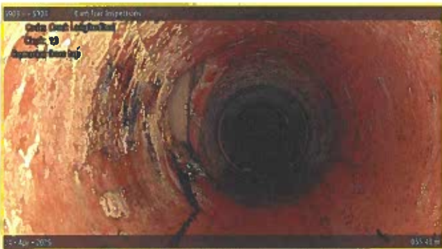
[Grade 2] Crack Longitudinal at 055.40 m, 10 o'clock | from tap
