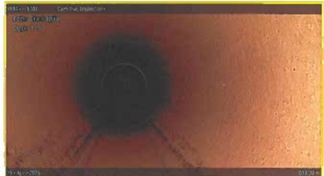
[Grade 2] Crack Spiral at 013.20 m, 3 - 5 o'clock
