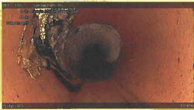
[Grade 2] Deposits Attached Encrustation at 021.80 m, 7 - 11 o'clock
