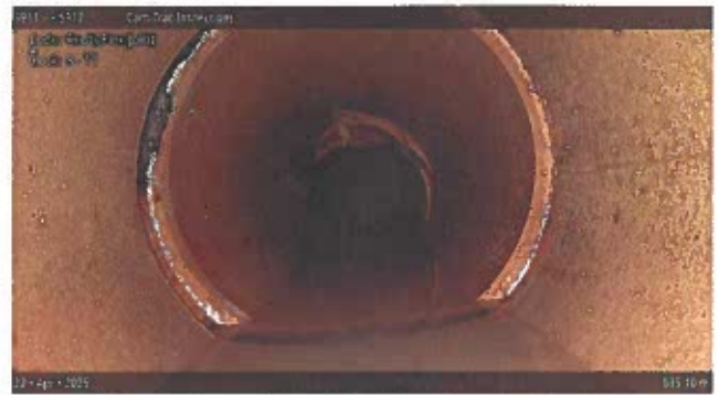
[Grade 1] Roots Fine Joint at 035.10 m, 8 - 11 o'clock
