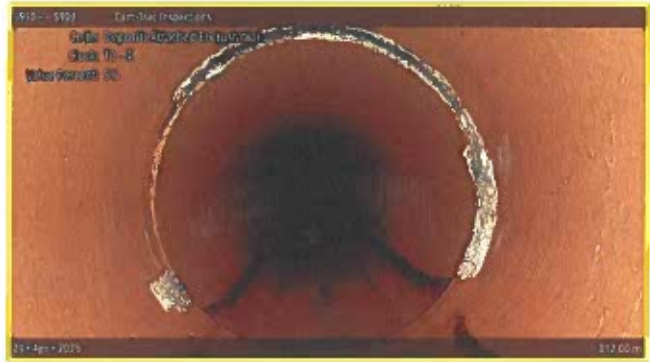
[Grade 2] Deposits Attached Encrustation at 012.00 m, 10 - 4 o'clock
