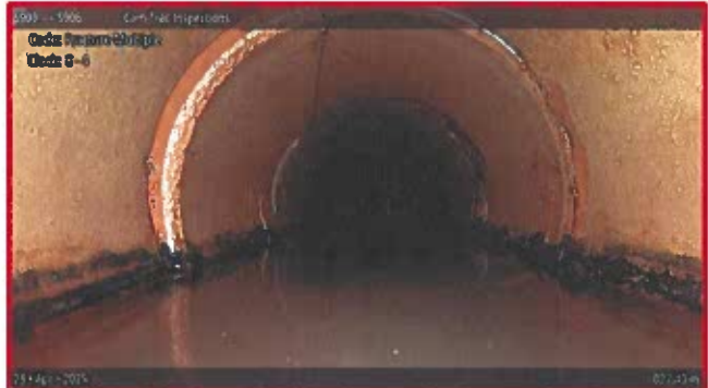
[Grade 4] Fracture Multiple at 027.40 m, 8 - 4 o'clock
