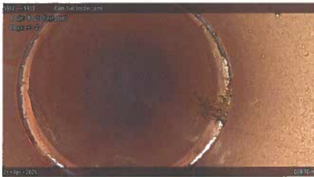
[Grade 1] Roots Fine Joint at 020.70 m, 8 - 4 o'clock
