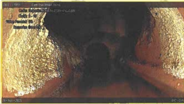
[Grade 2] Deposits Attached Encrustation at 092.80 m, 3 - 10 o'clock | from MH
