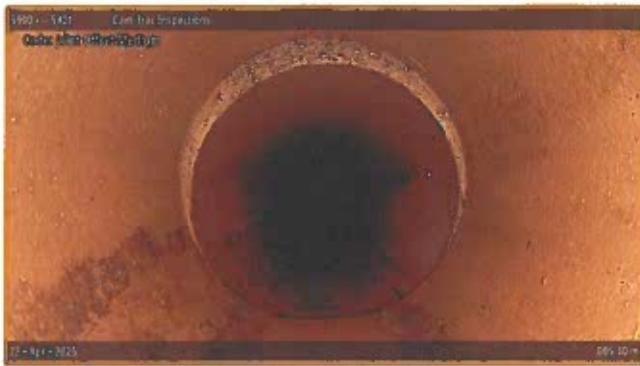
[Grade 3] Joint Offset Medium at 005.40 m
