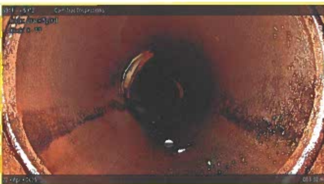
[Grade 2] Crack Spiral at 003.30 m, 8 - 11 o'clock
