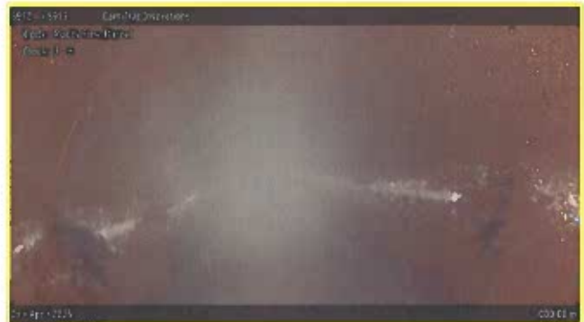
[Grade 2] Roots Fine Barrel at 000.00 m, 3 - 8 o'clock
