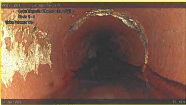
[Grade 2] Deposits Attached Encrustation at 021.60 m, 9 - 4 o'clock
