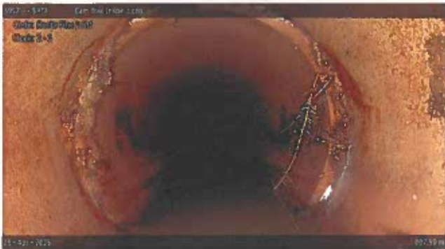
[Grade 1] Roots Fine Joint at 007.90 m, 2 - 5 o'clock
