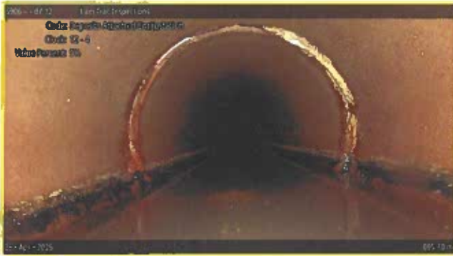
[Grade 2] Deposits Attached Encrustation at 005.80 m, 12 - 4 o'clock
