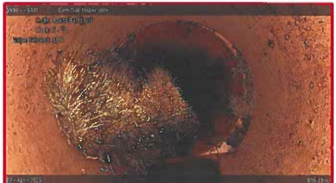
[Grade 4] Roots Ball Joint at 016.20 m, 5 - 10 o'clock
