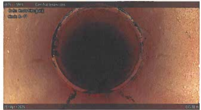
[Grade 1] Roots Fine Joint at 045.20 m, 8 - 11 o'clock
