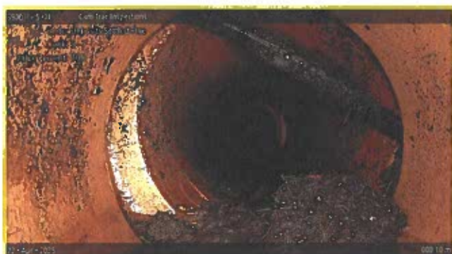
[Grade 2] Deposits Settled Fine at 000.10 m, 5 - 7 o'clock
