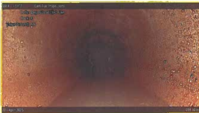
[Grade 2] Deposits Settled Fine at 038.10 m, 6 o'clock
