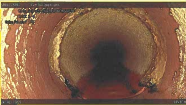
[Grade 2] Deposits Attached Encrustation at 065.50 m, 8 - 4 o'clock
