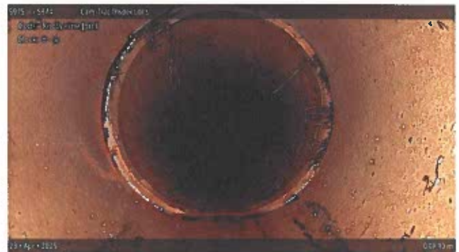
[Grade 1] Roots Fine Joint at 049.40 m, 8 - 4 o'clock
