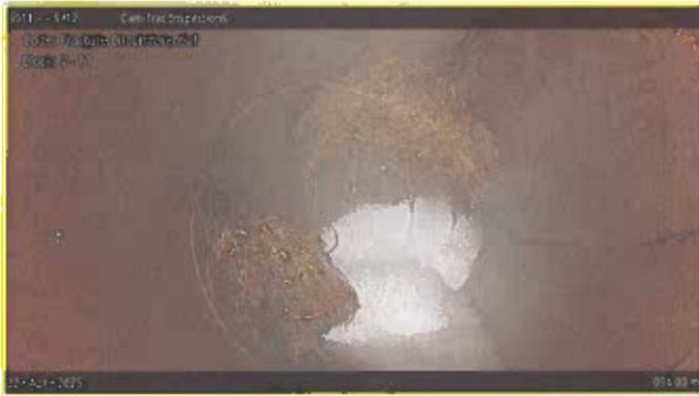
[Grade 2] Fracture Circumferential at 094.00 m, 7 - 11 o'clock
