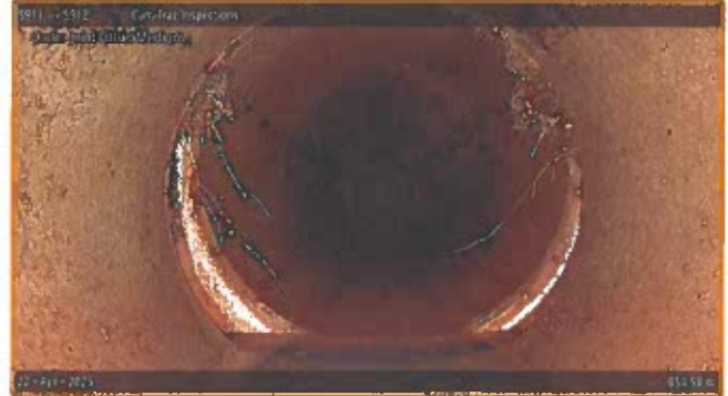
[Grade 3] Joint Offset Medium at 054.50 m
