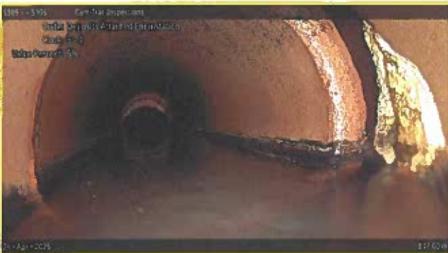
[Grade 2] Deposits Attached Encrustation at 047.00 m, 3 - 4 o'clock
