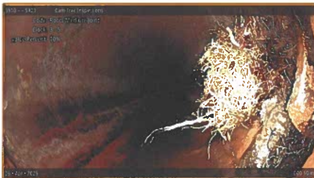
[Grade 3] Roots Medium Joint at 000.10 m, 3 - 5 o'clock
