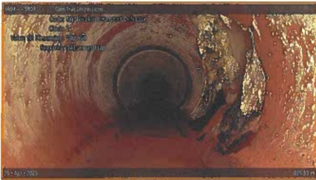
[Grade 3] Tap Break-in/Hammer Defective at 025.50 m, 2 o'clock | DAE around tap
