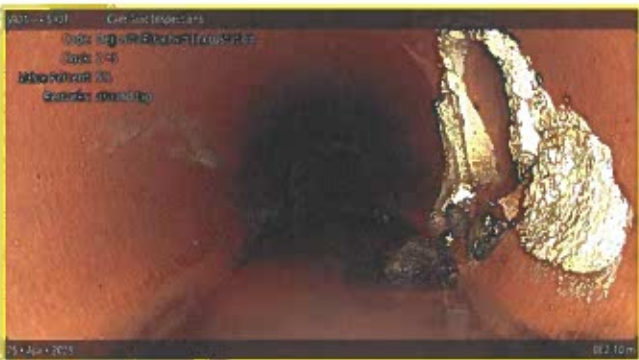
[Grade 2] Deposits Attached Encrustation at 062.10 m, 2 - 6 o'clock | around tap
