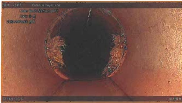
[Grade 3] Roots Medium Joint at 068.30 m, 8 - 4 o'clock
