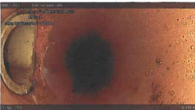
Tap Break-in/Hammer at 010.00 m, 9 o'clock
