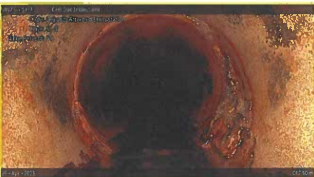
[Grade 2] Deposits Attached Encrustation at 017.50 m, 8 - 4 o'clock
