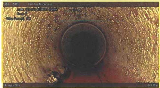
[Grade 2] Deposits Attached Encrustation at 084.70 m, 7 o'clock
