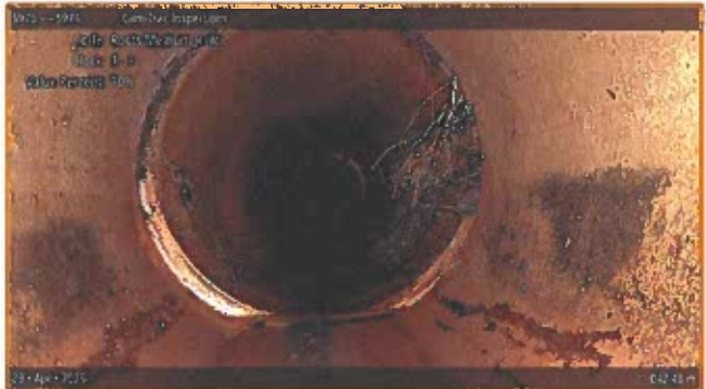
[Grade 3] Roots Medium Joint at 042.40 m, 9 - 3 o'clock
