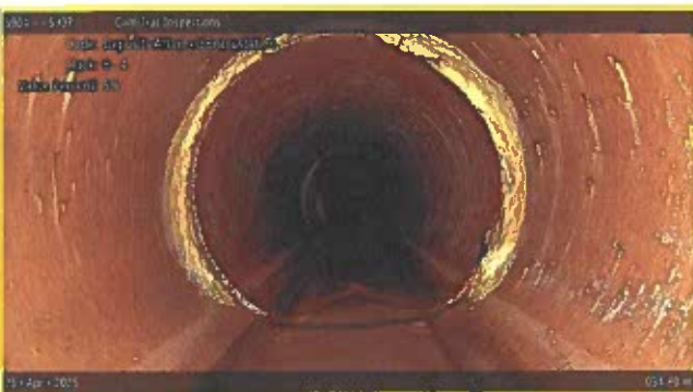
[Grade 2] Deposits Attached Encrustation at 054.80 m, 8 - 4 o'clock
