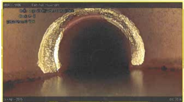
[Grade 2] Deposits Attached Encrustation at 032.80 m, 8 - 4 o'clock
