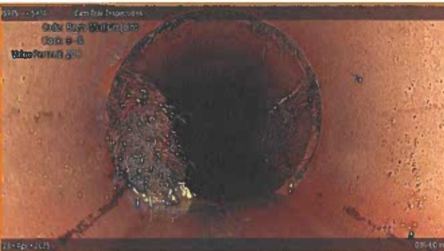
[Grade 3] Roots Medium Joint at 046.60 m, 8 - 4 o'clock
