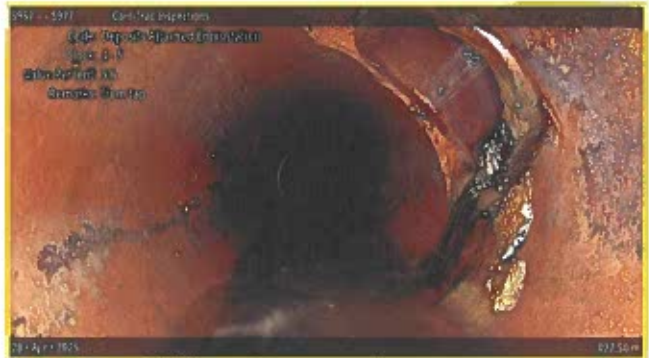
[Grade 2] Deposits Attached Encrustation at 027.50 m, 4 - 5 o'clock | from tap
