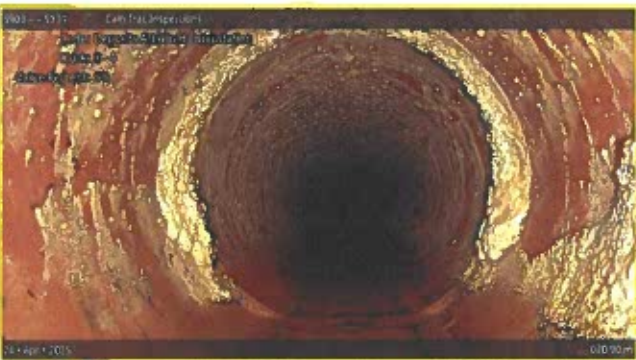
[Grade 2] Deposits Attached Encrustation at 020.90 m, 8 - 4 o'clock
