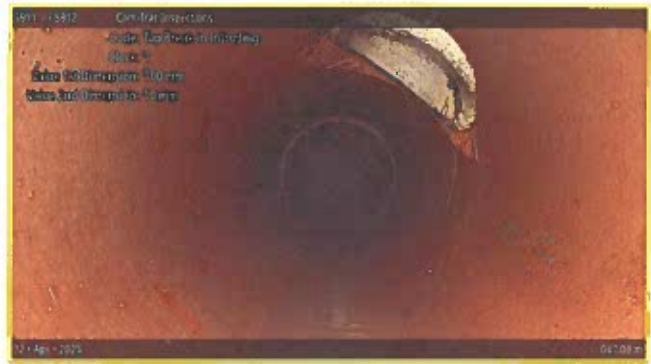
[Grade 2] Tap Break-in Intruding at 047.00 m, 1 o'clock
