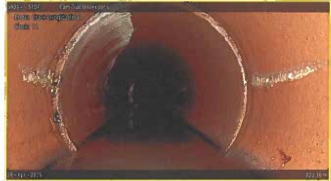
[Grade 2] Crack Longitudinal at 022.30 m, 11 o'clock
