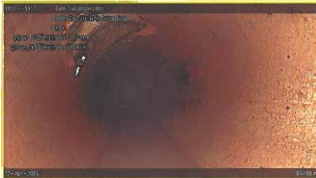
[Grade 2] Tap Break-in Intruding at 040.80 m, 10 o'clock
