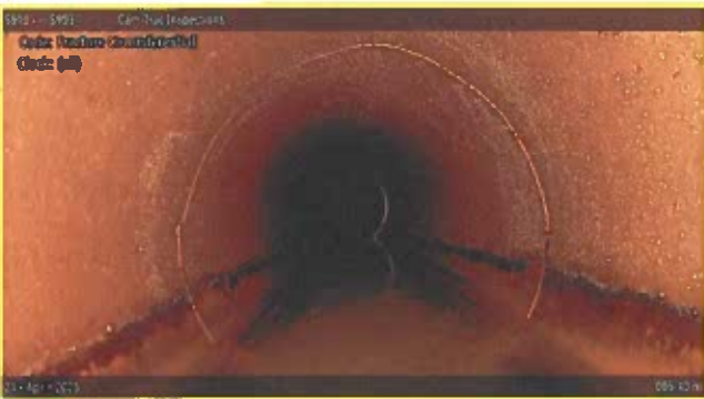
[Grade 2] Fracture Circumferential at 005.40 m, (all clock positions)
