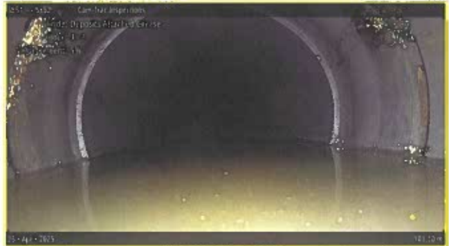
[Grade 2] Deposits Attached Grease at 101.10 m, 9 - 3 o'clock
