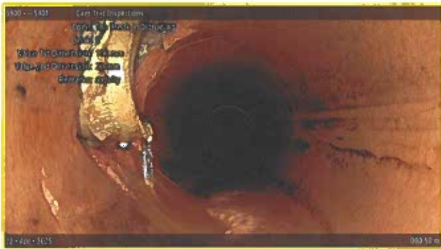
[Grade 2] Tap Break-in Intruding at 000.50 m, 9 o'clock | activity
