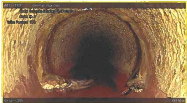
[Grade 2] Deposits Attached Encrustation at 062.80 m, 8 - 4 o'clock
