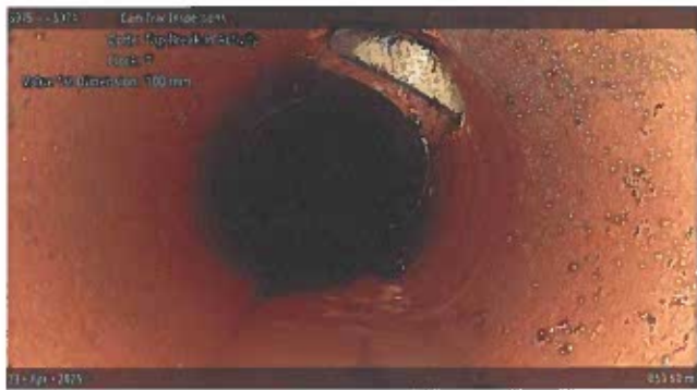
Tap Break-in Activity at 053.80 m, 1 o'clock
