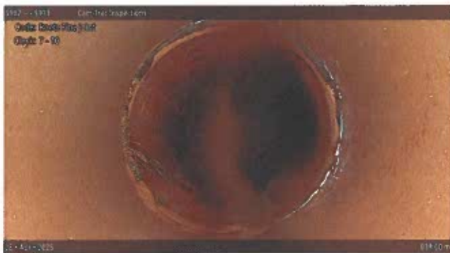
[Grade 1] Roots Fine Joint at 038.60 m, 7 - 10 o'clock
