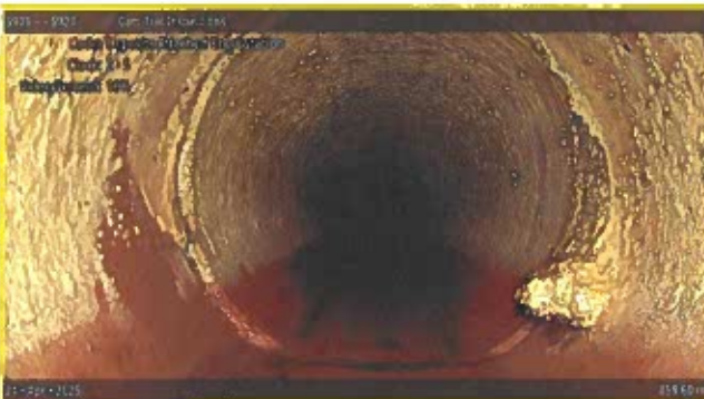
[Grade 2] Deposits Attached Encrustation at 058.60 m, 2 - 5 o'clock
