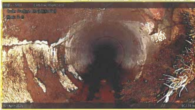
[Grade 2] Fracture Circumferential at 002.90 m, 4 - 8 o'clock
