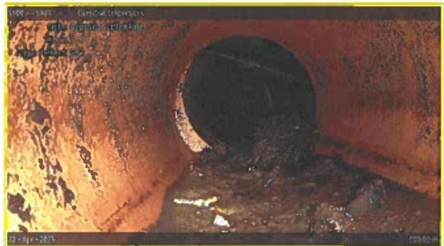
[Grade 2] Deposits Settled Fine at 000.00 m, 5 - 7 o'clock
