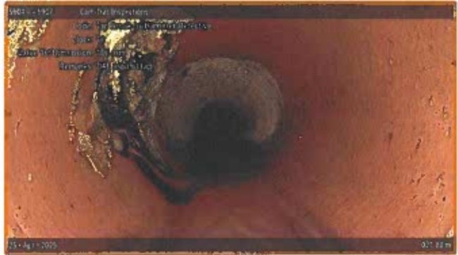
[Grade 3] Tap Break-in/Hammer Defective at 021.80 m, 10 o'clock | DAE around tap
