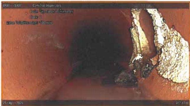
[Grade 3] Tap Break-in/Hammer Defective at 062.10 m, 3 o'clock | DAE around tap
