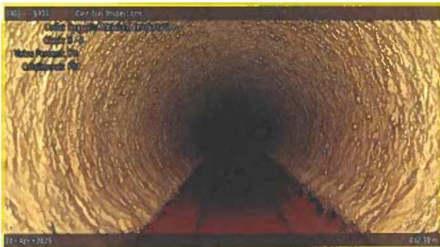
[Grade 2] Deposits Attached Encrustation (finish) at 042.30 m, 8 - 4 o'clock
