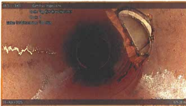
[Grade 3] Tap Break-in/Hammer Defective at 025.30 m, 2 o'clock | roots
