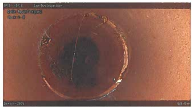
[Grade 1] Roots Fine Joint at 035.80 m, 8 - 4 o'clock
