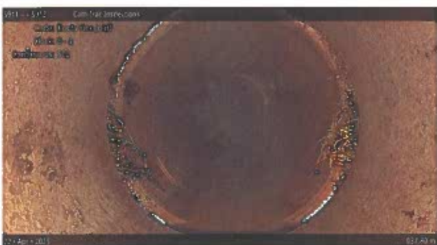
[Grade 1] Roots Fine Joint at 087.80 m, 8 - 4 o'clock
