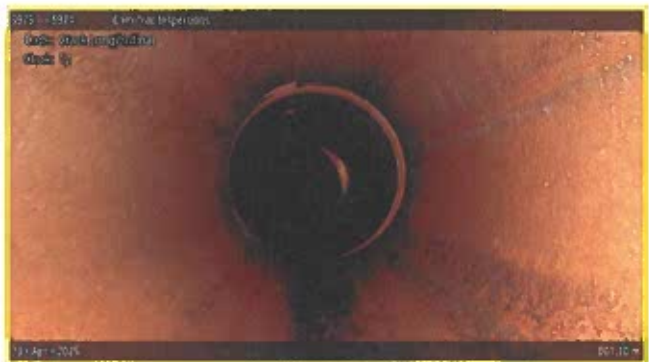
[Grade 2] Crack Longitudinal at 001.10 m, 12 o'clock
