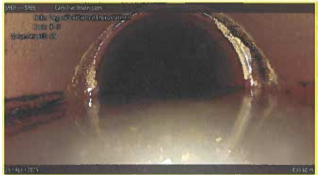
[Grade 2] Deposits Attached Encrustation at 035.60 m, 9 - 3 o'clock
