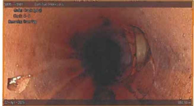
[Grade 3] Fracture Spiral at 002.80 m, 4 - 5 o'clock | from tap
