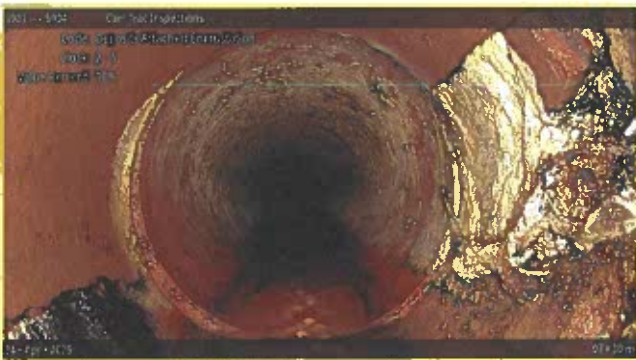
[Grade 2] Deposits Attached Encrustation at 079.30 m, 2 - 5 o'clock
