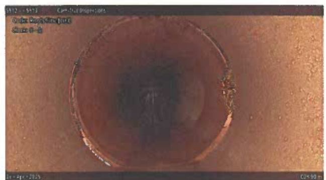
[Grade 1] Roots Fine Joint at 028.90 m, 8 - 4 o'clock
