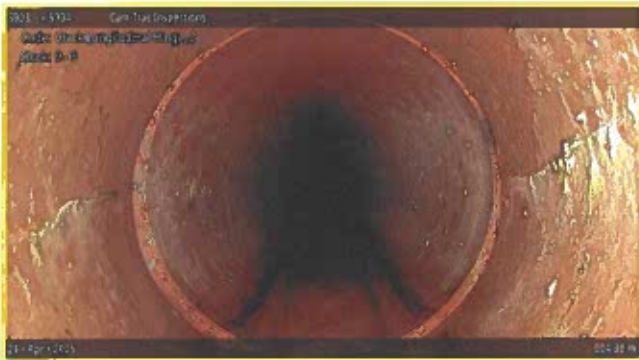
[Grade 2] Crack Longitudinal Hinge, 2 at 004.30 m, 9 - 3 o'clock
