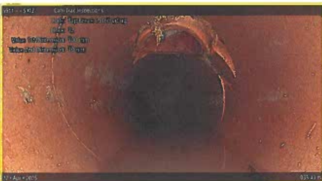
[Grade 2] Tap Break-in Intruding at 035.40 m, 12 o'clock
