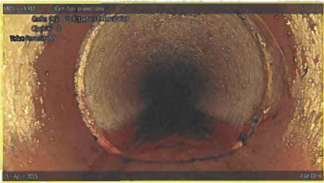
[Grade 2] Deposits Attached Encrustation at 030.00 m, 1 - 4 o'clock
