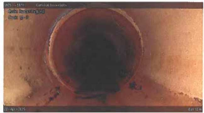
[Grade 1] Roots Fine Joint at 034.10 m, 12 - 3 o'clock
