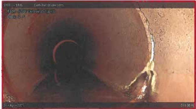
[Grade 5] Infiltration Gusher Joint at 043.30 m, 4 - 5 o'clock
