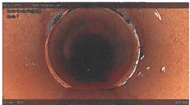
[Grade 1] Roots Fine Joint at 073.10 m, 1 o'clock
