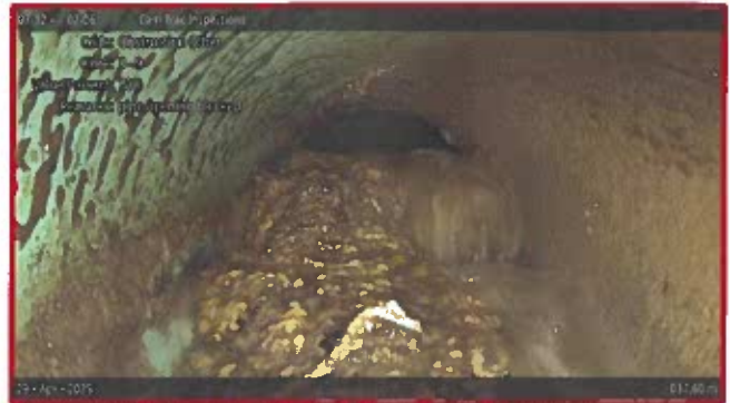
[Grade 5] Obstruction Other at 037.60 m, 3 - 9 o'clock | pipe opening blocked
