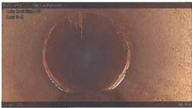
[Grade 1] Roots Fine Joint at 006.80 m, 9 - 4 o'clock
