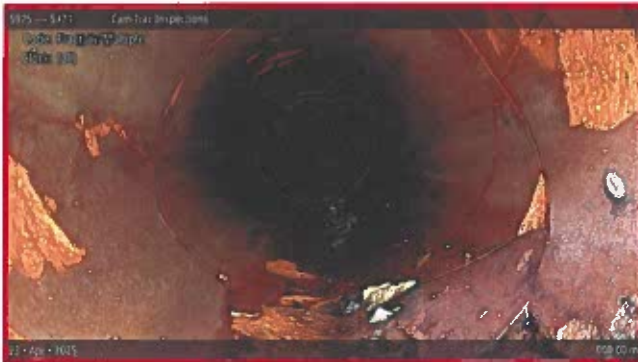
[Grade 4] Fracture Multiple at 000.00 m, (all clock positions)
