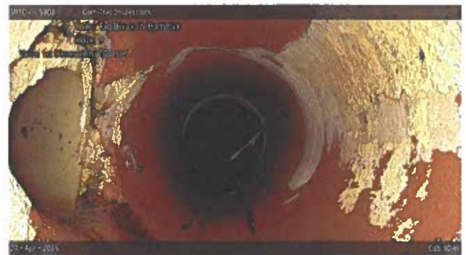
Tap Break-in/Hammer at 036.30 m, 9 o'clock
