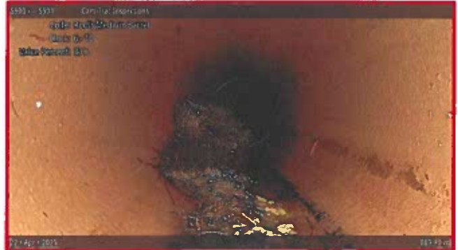
[Grade 4] Roots Medium Barrel at 069.80 m, 6 - 10 o'clock
