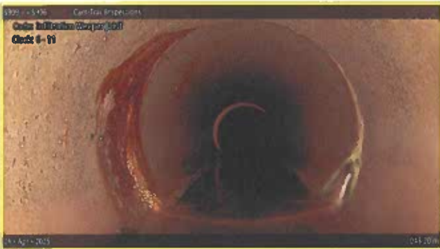
[Grade 2] Infiltration Weeper Joint at 043.20 m, 6 - 11 o'clock
