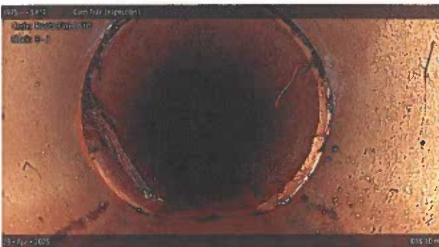
[Grade 1] Roots Fine Joint at 048.10 m, 8 - 3 o'clock
