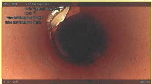
[Grade 2] Tap Break-in Intruding at 058.30 m, 11 o'clock
