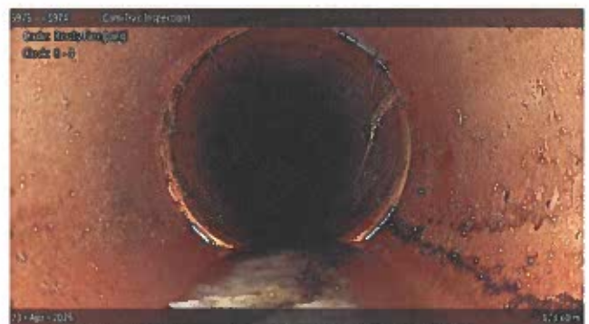
[Grade 1] Roots Fine Joint at 028.60 m, 8 - 4 o'clock
