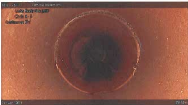
[Grade 1] Roots Fine Joint (finish) at 059.50 m, 8 - 4 o'clock
