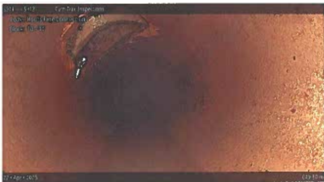
[Grade 1] Roots Fine Connection at 040.80 m, 10 - 11 o'clock
