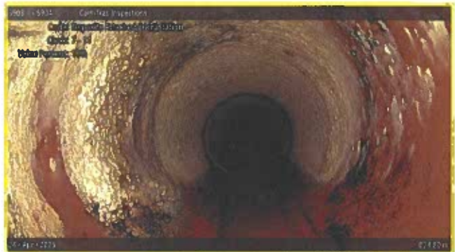
[Grade 2] Deposits Attached Encrustation at 028.80 m, 7 - 11 o'clock
