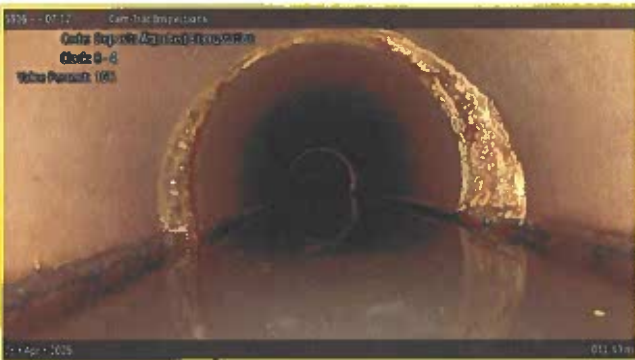
[Grade 2] Deposits Attached Encrustation at 011.40 m, 8 - 4 o'clock
