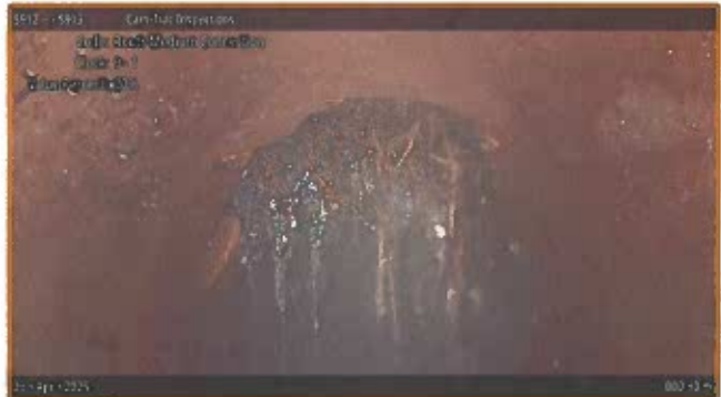
[Grade 3] Roots Medium Connection at 000.80 m, 9 - 1 o'clock
