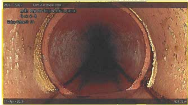
[Grade 2] Deposits Attached Encrustation at 005.70 m, 8 - 4 o'clock
