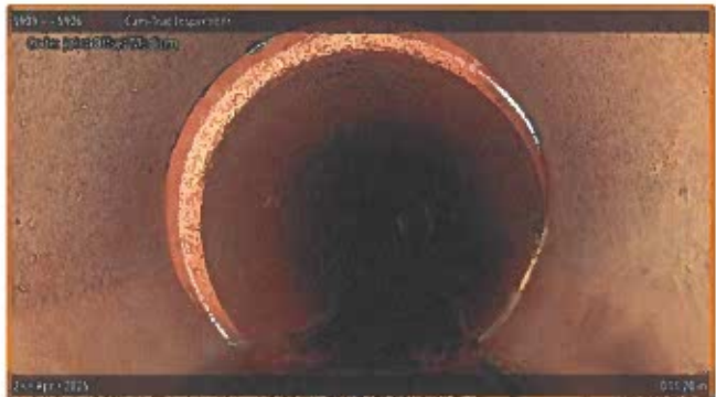
[Grade 3] Joint Offset Medium at 044.20 m
