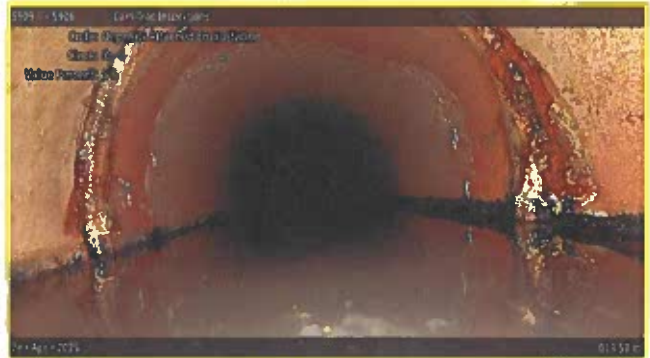
[Grade 2] Deposits Attached Encrustation at 013.50 m, 8 - 4 o'clock
