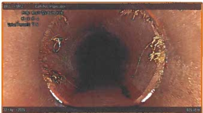
[Grade 3] Roots Medium Joint at 075.40 m, 8 - 4 o'clock
