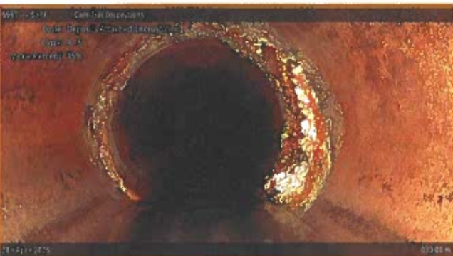
[Grade 3] Deposits Attached Encrustation at 030.00 m, 9 - 5 o'clock
