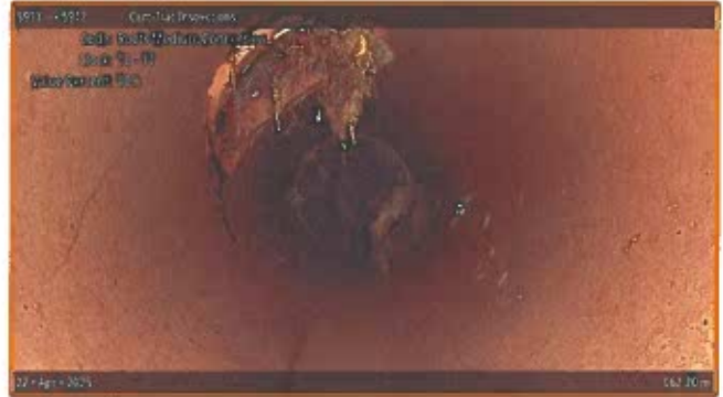
[Grade 3] Roots Medium Connection at 062.20 m, 10 - 11 o'clock
