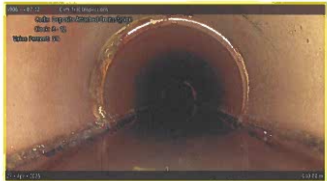
[Grade 2] Deposits Attached Encrustation at 010.00 m, 8 - 12 o'clock
