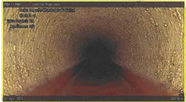
[Grade 2] Deposits Attached Encrustation (start) at 002.50 m, 8 - 4 o'clock
