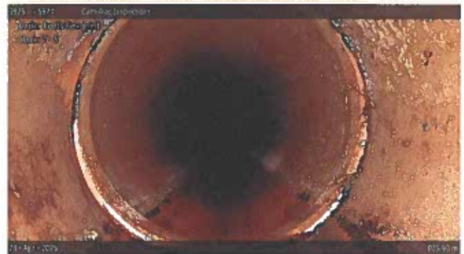
[Grade 1] Roots Fine Joint at 025.90 m, 1 - 5 o'clock
