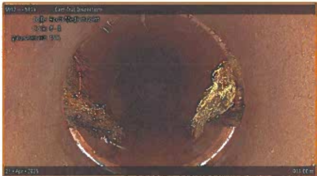
[Grade 3] Roots Medium Joint at 011.00 m, 8 - 4 o'clock
