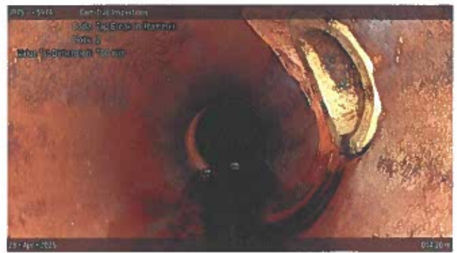
Tap Break-in/Hammer at 014.20 m, 2 o'clock
