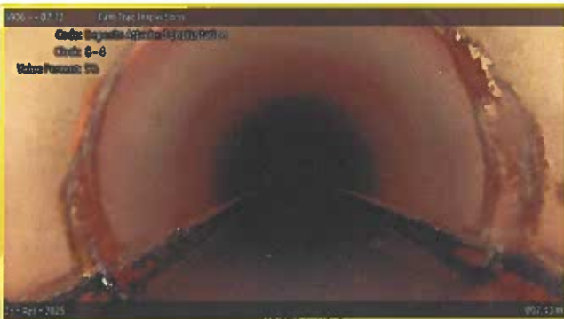
[Grade 2] Deposits Attached Encrustation at 007.30 m, 8 - 4 o'clock
