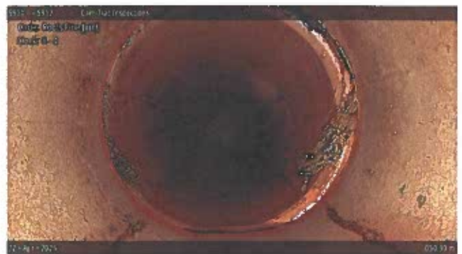
[Grade 1] Roots Fine Joint at 050.30 m, 8 - 4 o'clock
