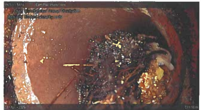
Miscellaneous General Observation at 083.10 m | blocked Lateral by roots
