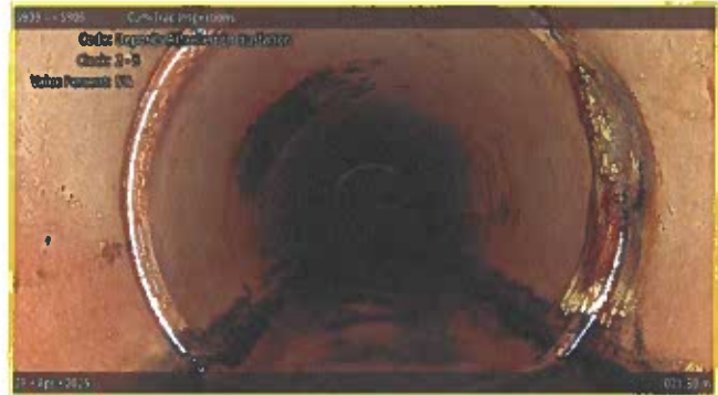
[Grade 2] Deposits Attached Encrustation at 021.80 m, 2 - 5 o'clock
