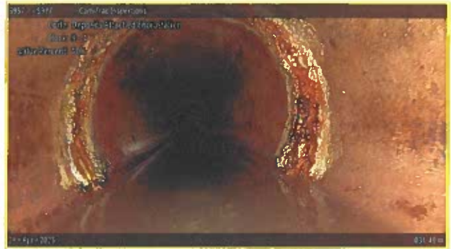
[Grade 2] Deposits Attached Encrustation at 031.40 m, 8 - 4 o'clock
