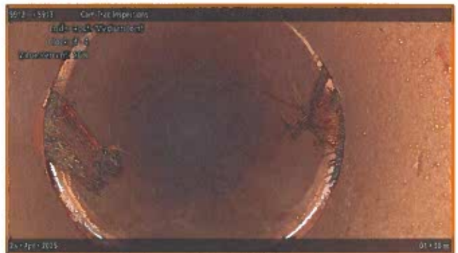
[Grade 3] Roots Medium Joint at 019.30 m, 8 - 4 o'clock
