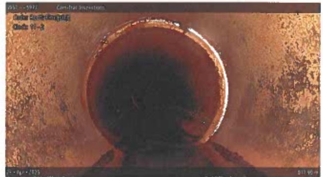
[Grade 1] Roots Fine Joint at 011.90 m, 11 - 2 o'clock
