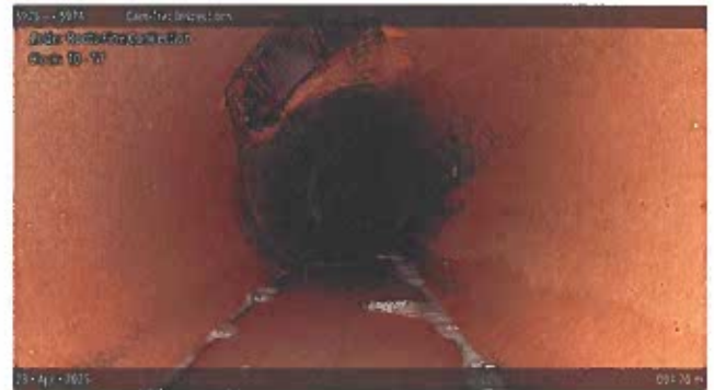
[Grade 1] Roots Fine Connection at 094.70 m, 10 - 11 o'clock
