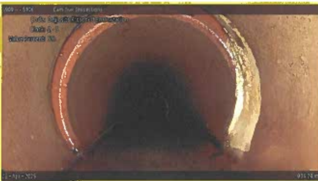
[Grade 2] Deposits Attached Encrustation at 034.20 m, 2 - 5 o'clock
