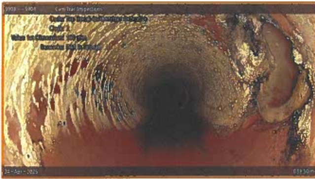
[Grade 3] Tap Break-in/Hammer Defective at 039.50 m, 2 o'clock | DAE in lateral
