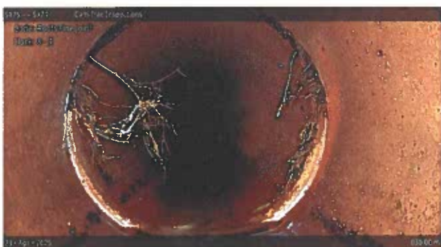
[Grade 1] Roots Fine Joint at 030.00 m, 8 - 4 o'clock
