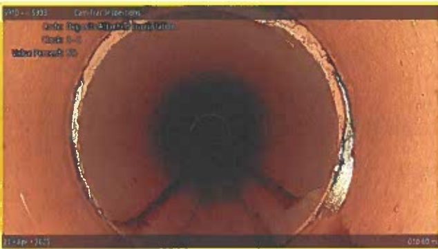
[Grade 2] Deposits Attached Encrustation at 010.60 m, 3 - 5 o'clock
