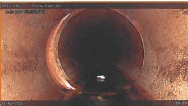
[Grade 3] Joint Offset Medium at 014.70 m
