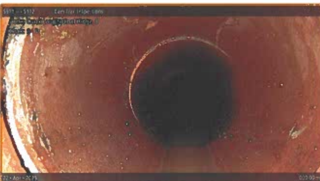
[Grade 3] Crack Longitudinal Hinge, 3 at 000.00 m, 9 - 3 o'clock
