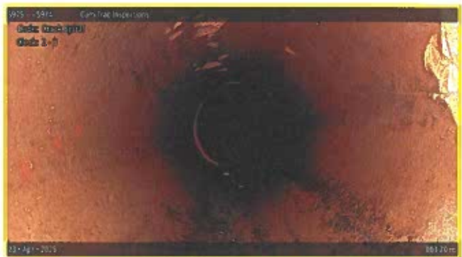
[Grade 2] Crack Spiral at 003.20 m, 2 - 3 o'clock
