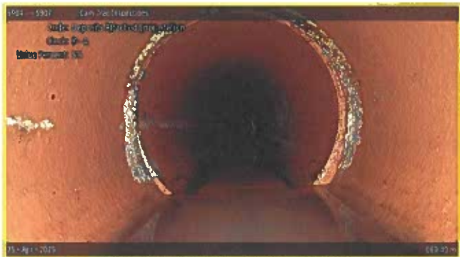
[Grade 2] Deposits Attached Encrustation at 060.40 m, 8 - 4 o'clock
