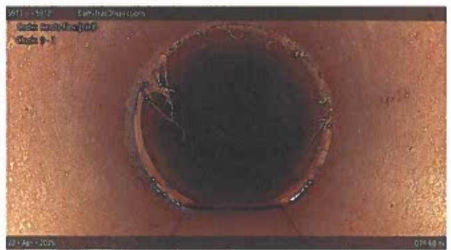
[Grade 1] Roots Fine Joint at 078.10 m, 9 - 5 o'clock
