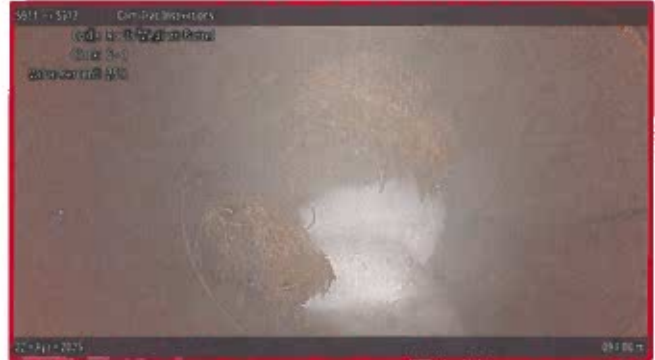
[Grade 4] Roots Medium Barrel at 094.00 m, 6 - 1 o'clock
