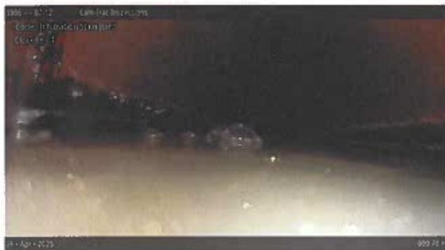
[Grade 1] Infiltration Stain Joint at 000.70 m, 8 - 4 o'clock
