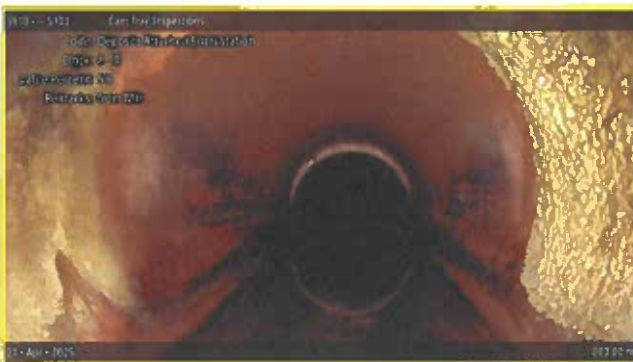
[Grade 2] Deposits Attached Encrustation at 000.00 m, 8 - 4 o'clock | from MH
