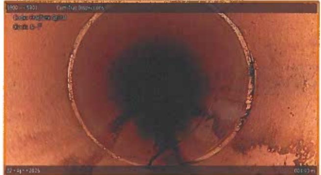
[Grade 3] Fracture Spiral at 003.90 m, 4 - 7 o'clock
