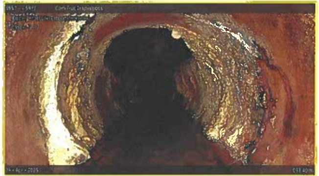
[Grade 2] Fracture Circumferential at 033.40 m, 5 - 7 o'clock
