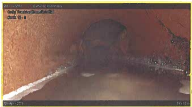
[Grade 2] Fracture Circumferential at 095.40 m, 12 - 5 o'clock
