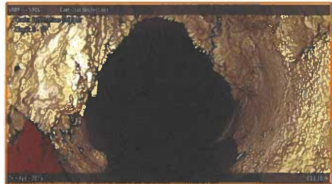
[Grade 3] Infiltration Dripper at 000.10 m, 8 - 11 o'clock
