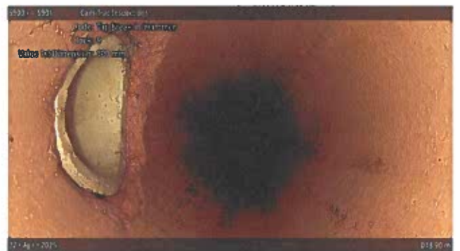
Tap Break-in/Hammer at 048.90 m, 9 o'clock
