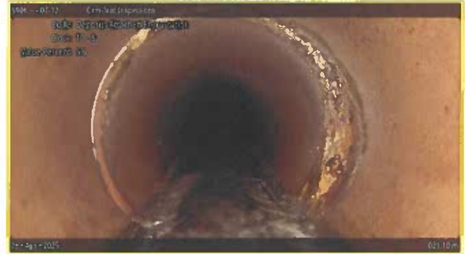
[Grade 2] Deposits Attached Encrustation at 021.10 m, 10 - 5 o'clock
