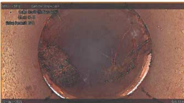
[Grade 3] Roots Medium Joint at 086.40 m, 8 - 4 o'clock
