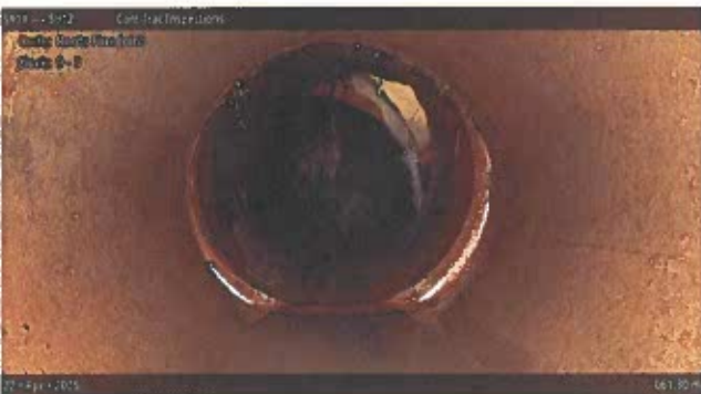
[Grade 1] Roots Fine Joint at 061.30 m, 9 - 3 o'clock
