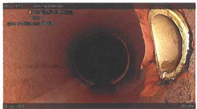
Tap Break-in Activity at 004.30 m, 3 o'clock
