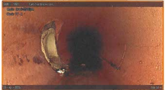
[Grade 3] Crack Multiple at 066.50 m, 11 - 5 o'clock
