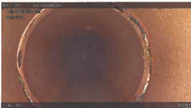
[Grade 1] Roots Fine Joint at 023.50 m, 8 - 4 o'clock
