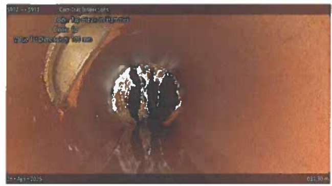
Tap Break-in/Hammer at 031.30 m, 10 o'clock
