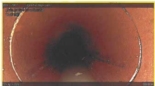
[Grade 2] Fracture Circumferential at 000.00 m, (all clock positions)
