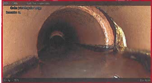
[Grade 4] Joint Angular Large at 046.90 m | LL
