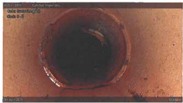
[Grade 1] Roots Fine Joint at 053.60 m, 8 - 4 o'clock
