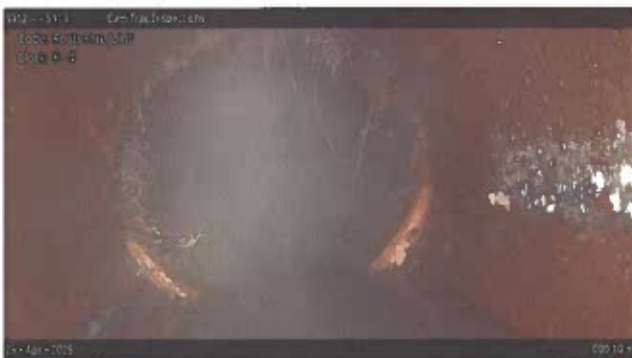
[Grade 1] Roots Fine Joint at 000.10 m, 8 - 4 o'clock
