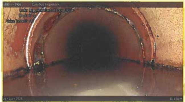
[Grade 2] Deposits Attached Encrustation at 014.90 m, 8 - 4 o'clock
