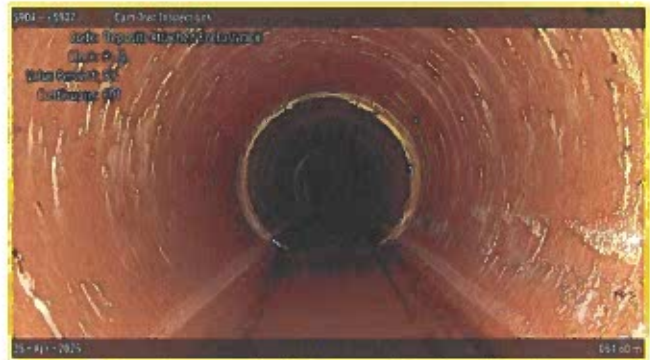
[Grade 2] Deposits Attached Encrustation (finish) at 054.60 m, 8 - 4 o'clock
