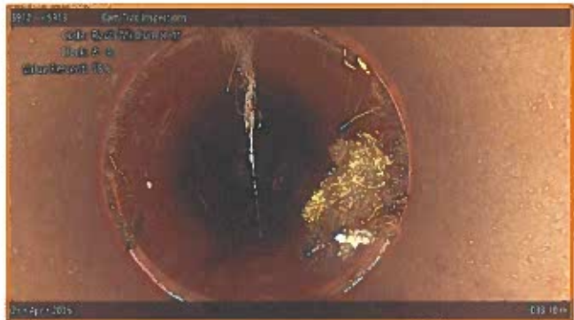
[Grade 3] Roots Medium Joint at 033.10 m, 8 - 4 o'clock
