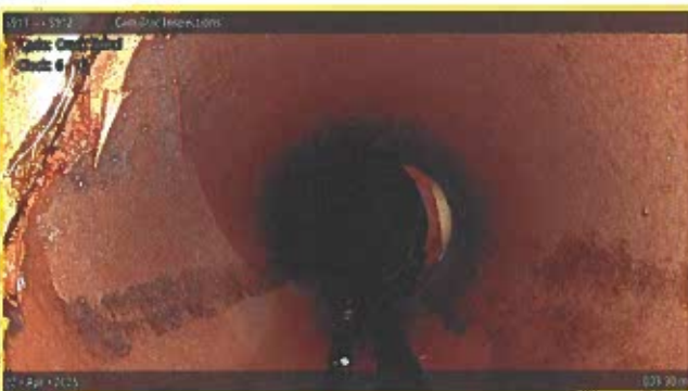
[Grade 2] Crack Spiral at 003.90 m, 6 - 10 o'clock
