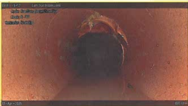
[Grade 2] Fracture Circumferential at 035.40 m, 6 - 11 o'clock | from tap
