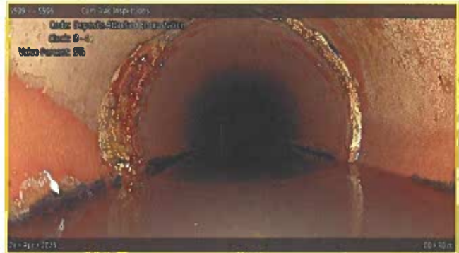
[Grade 2] Deposits Attached Encrustation at 009.30 m, 8 - 4 o'clock
