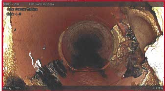
[Grade 4] Fracture Multiple at 079.20 m, 4 - 8 o'clock
