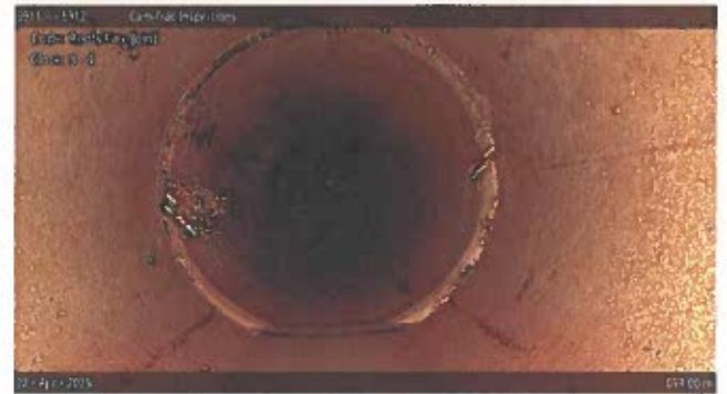
[Grade 1] Roots Fine Joint at 057.60 m, 8 - 4 o'clock
