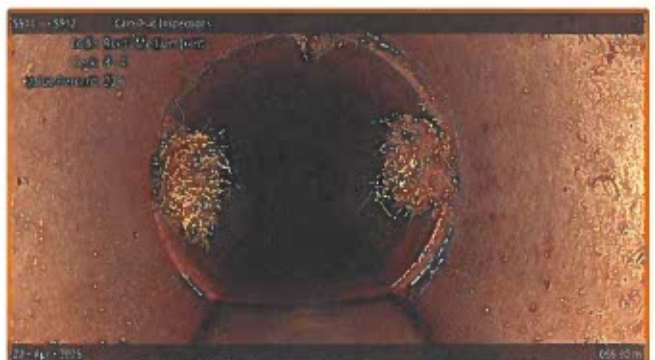
[Grade 3] Roots Medium Joint at 066.90 m, 8 - 4 o'clock
