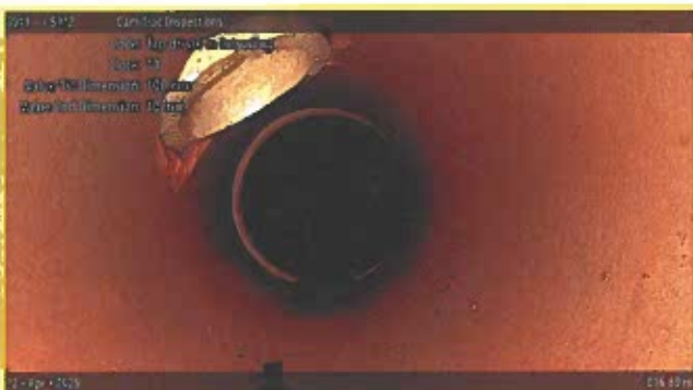
[Grade 2] Tap Break-in Intruding at 016.80 m, 11 o'clock
