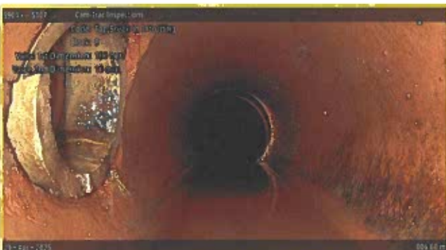
[Grade 2] Tap Break-in Intruding at 006.60 m, 9 o'clock
