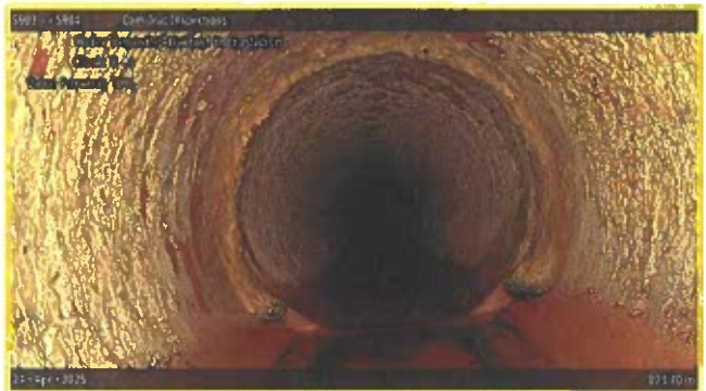
[Grade 2] Deposits Attached Encrustation at 023.70 m, 8 - 4 o'clock
