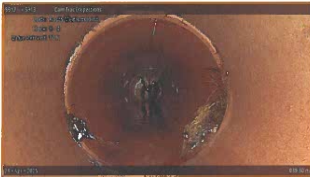
[Grade 3] Roots Medium Joint at 030.30 m, 8 - 4 o'clock
