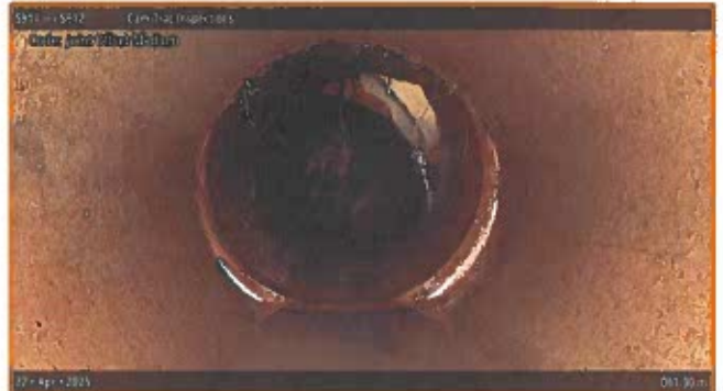
[Grade 3] Joint Offset Medium at 061.30 m
