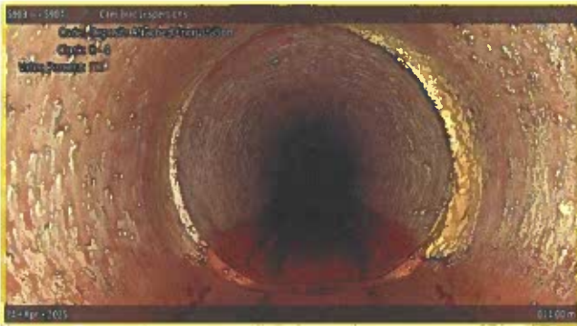
[Grade 2] Deposits Attached Encrustation at 014.00 m, 8 - 4 o'clock
