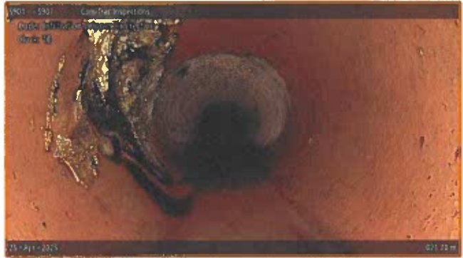
[Grade 3] Infiltration Dripper Connection at 021.80 m, 10 o'clock
