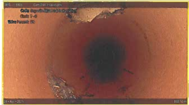
[Grade 2] Deposits Attached Encrustation at 032.90 m, 7 - 8 o'clock
