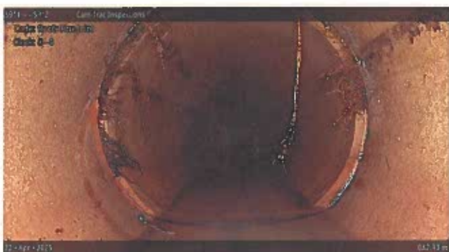
[Grade 1] Roots Fine Joint at 082.30 m, 8 - 4 o'clock
