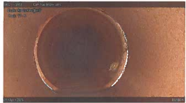
[Grade 1] Roots Fine Joint at 022.00 m, 11 - 5 o'clock
