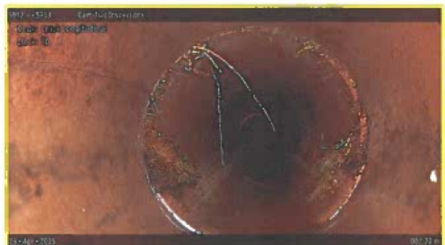
[Grade 2] Crack Longitudinal at 002.70 m, 10 o'clock
