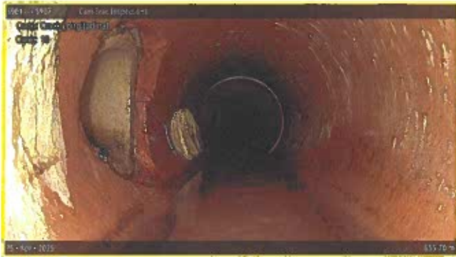
[Grade 2] Crack Longitudinal at 055.70 m, 10 o'clock
