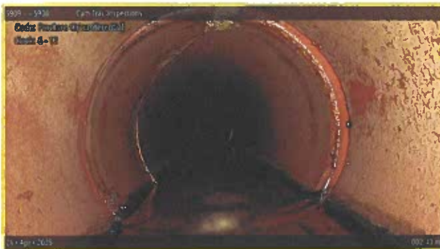
[Grade 2] Fracture Circumferential at 002.40 m, 6 - 12 o'clock
