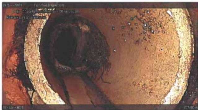
Miscellaneous General Observation at 025.60 m | roots in lateral
