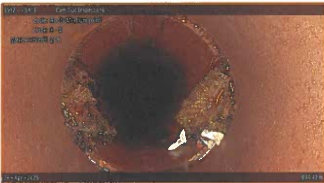
[Grade 3] Roots Medium Joint at 034.40 m, 8 - 4 o'clock
