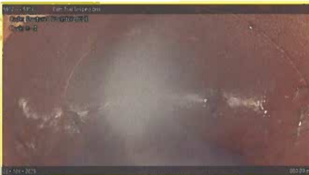
[Grade 2] Fracture Circumferential at 000.00 m, 8 - 4 o'clock
