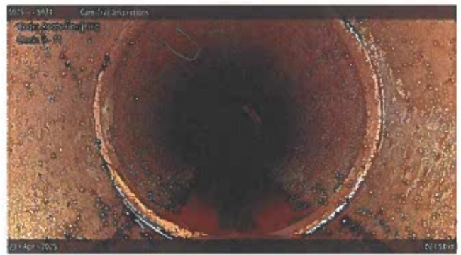
[Grade 1] Roots Fine Joint at 024.50 m, 9 - 11 o'clock
