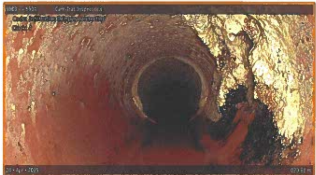
[Grade 3] Infiltration Dripper Connection at 020.60 m, 1 o'clock
