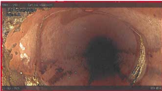
[Grade 4] Fracture Multiple at 000.00 m, 8 - 4 o'clock
