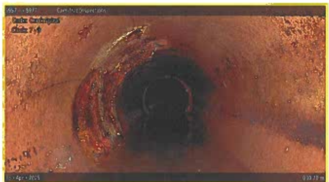
[Grade 2] Crack Spiral at 030.70 m, 7 - 9 o'clock
