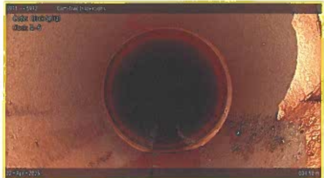
[Grade 2] Crack Spiral at 004.50 m, 4 - 6 o'clock
