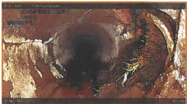
[Grade 3] Roots Medium Connection at 002.80 m, 2 - 4 o'clock
