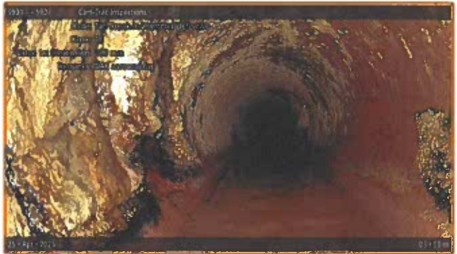
[Grade 3] Tap Break-in/Hammer Defective at 039.80 m, 10 o'clock | DAE around tap
