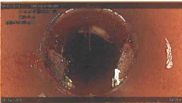
[Grade 3] Roots Medium Joint at 037.20 m, 8 - 4 o'clock
