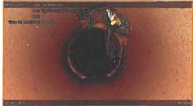
[Grade 3] Tap Break-in/Hammer Defective at 082.60 m, 1 o'clock | roots around tap and in lateral
