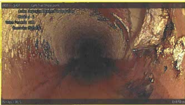
[Grade 2] Deposits Attached Encrustation at 040.50 m, 4 - 5 o'clock | from tap
