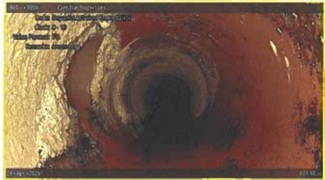
[Grade 2] Deposits Attached Encrustation at 028.50 m, 8 - 10 o'clock | around tap
