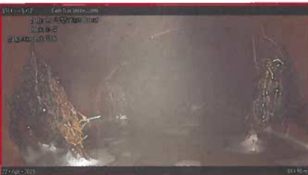
[Grade 4] Roots Medium Barrel at 094.90 m, 8 - 4 o'clock
