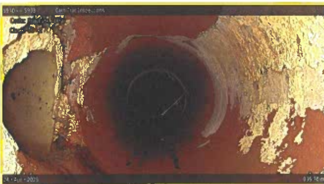
[Grade 2] Crack Spiral at 036.30 m, 10 - 2 o'clock
