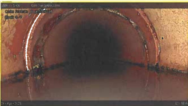
[Grade 2] Fracture Circumferential at 014.90 m, 4 - 6 o'clock
