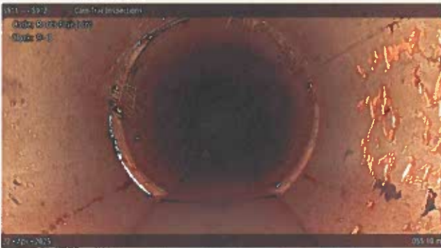
[Grade 1] Roots Fine Joint at 055.80 m, 9 - 3 o'clock
