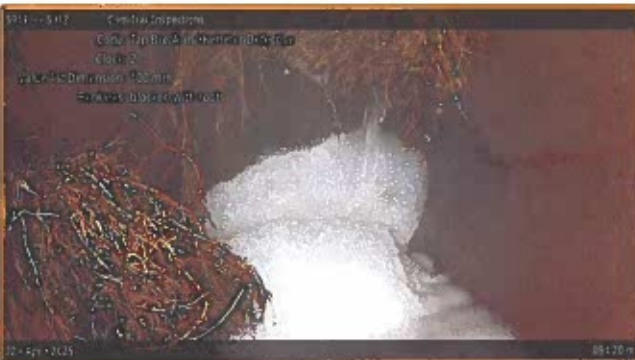
[Grade 3] Tap Break-in/Hammer Defective at 094.20 m, 2 o'clock | blocked with roots; activity
