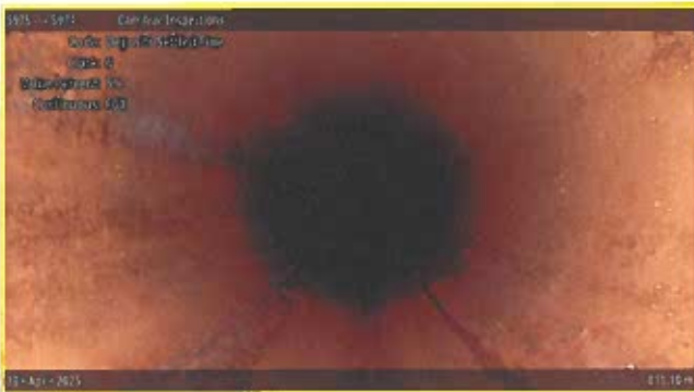
[Grade 2] Deposits Settled Fine (finish) at 011.10 m, 6 o'clock
