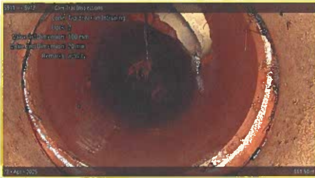
[Grade 2] Tap Break-in Intruding at 061.50 m, 2 o'clock | activity
