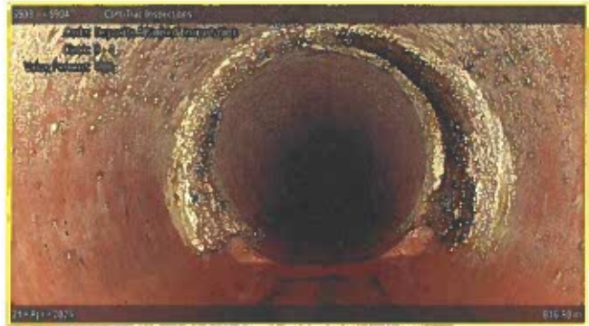
[Grade 2] Deposits Attached Encrustation at 016.80 m, 8 - 4 o'clock
