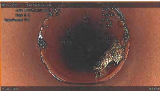
[Grade 3] Roots Medium Joint at 062.80 m, 8 - 4 o'clock
