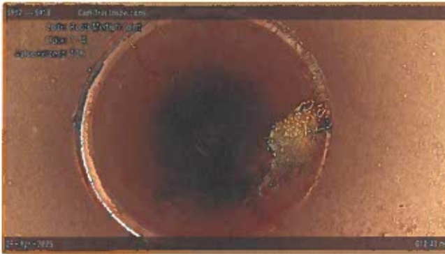
[Grade 3] Roots Medium Joint at 012.40 m, 1 - 4 o'clock
