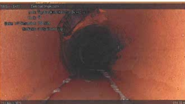
[Grade 3] Tap Break-in/Hammer Defective at 094.70 m, 10 o'clock | roots around tap
