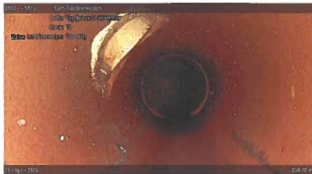
Tap Break-in/Hammer at 050.70 m, 10 o'clock
