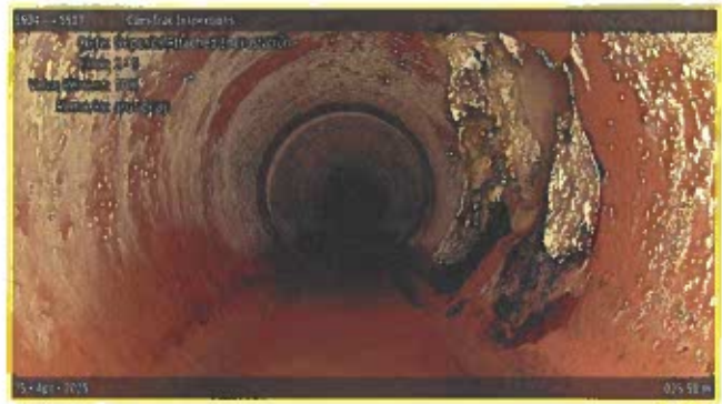
[Grade 2] Deposits Attached Encrustation at 025.50 m, 2 - 5 o'clock | around tap
