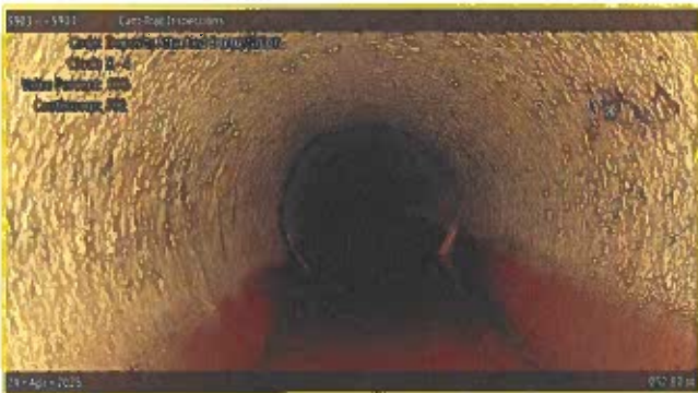
[Grade 2] Deposits Attached Encrustation (finish) at 052.80 m, 8 - 4 o'clock
