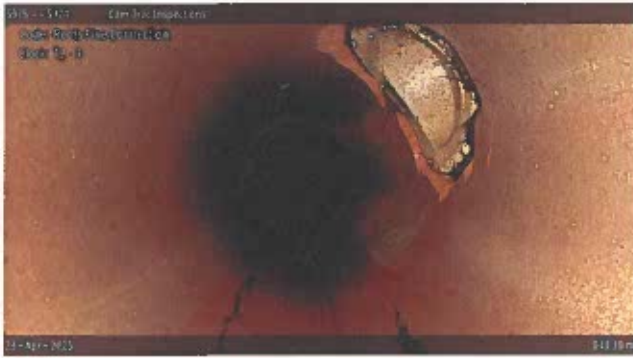
[Grade 1] Roots Fine Connection at 043.30 m, 12 - 3 o'clock
