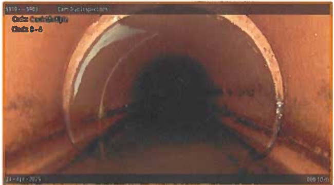
[Grade 3] Crack Multiple at 000.10 m, 8 - 4 o'clock
