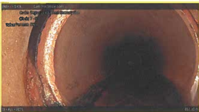
[Grade 2] Deposits Attached Encrustation at 051.30 m, 7 - 8 o'clock
