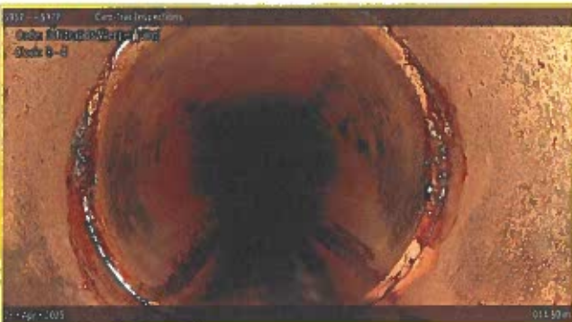
[Grade 2] Infiltration Weeper Joint at 014.80 m, 8 - 4 o'clock
