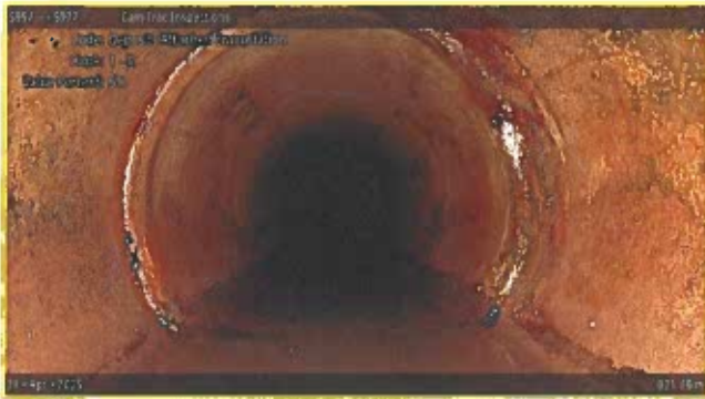
[Grade 2] Deposits Attached Encrustation at 021.80 m, 1 - 4 o'clock
