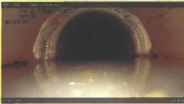
[Grade 2] Deposits Attached Encrustation at 037.00 m, 8 - 4 o'clock
