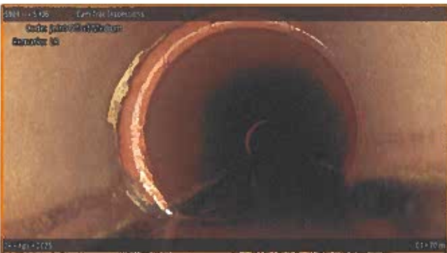
[Grade 3] Joint Offset Medium at 049.70 m | LR
