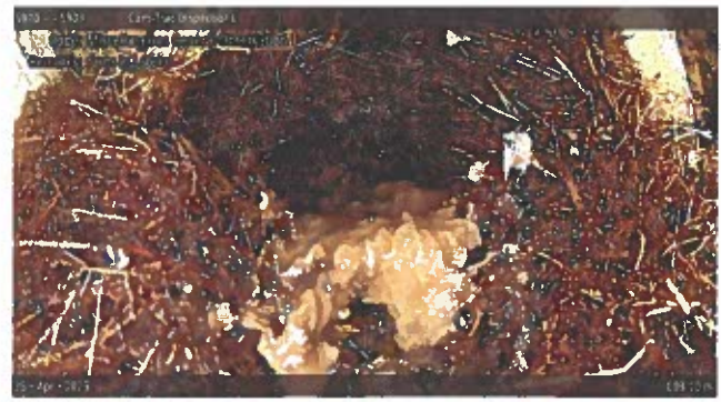
Miscellaneous General Observation at 003.10 m | roots in Lateral
