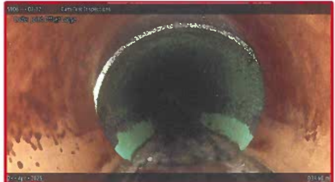
[Grade 4] Joint Offset Large at 033.60 m
