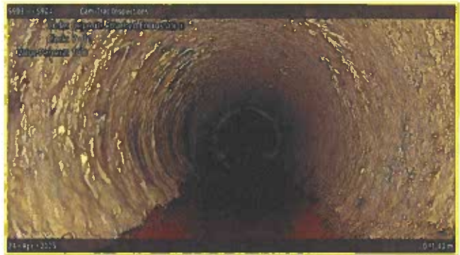
[Grade 2] Deposits Attached Encrustation at 031.40 m, 7 - 11 o'clock
