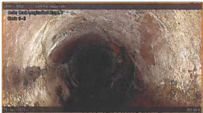
[Grade 3] Crack Longitudinal Hinge, 3 at 002.60 m, 9 - 3 o'clock
