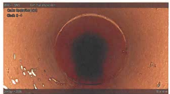
[Grade 1] Roots Fine Joint at 038.10 m, 8 - 4 o'clock
