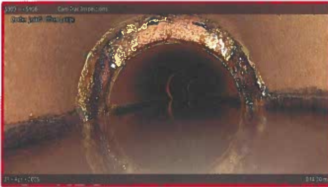
[Grade 4] Joint Offset Large at 048.20 m
