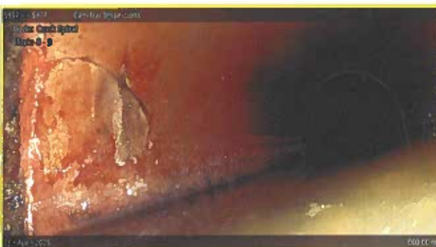
[Grade 2] Crack Spiral at 000.00 m, 8 - 9 o'clock
