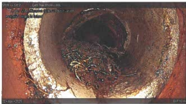
Miscellaneous General Observation at 047.40 m | roots in lateral
