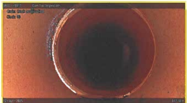
[Grade 2] Crack Longitudinal at 017.10 m, 10 o'clock
