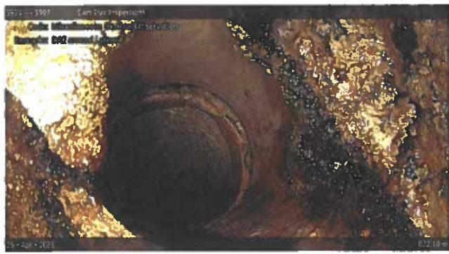
Miscellaneous General Observation at 022.10 m | DAE around Lateral
