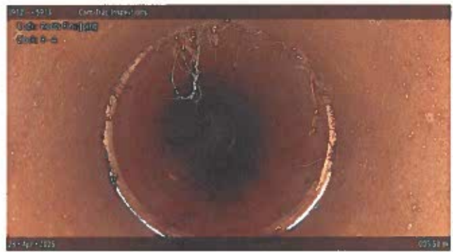
[Grade 1] Roots Fine Joint at 005.50 m, 8 - 4 o'clock
