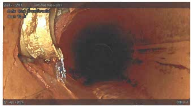
[Grade 1] Crack Circumferential at 000.60 m, 10 - 5 o'clock
