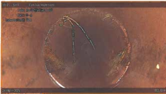
[Grade 3] Roots Medium Joint at 002.70 m, 8 - 4 o'clock
