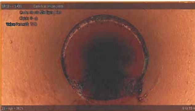
[Grade 3] Roots Medium Joint at 040.90 m, 8 - 4 o'clock
