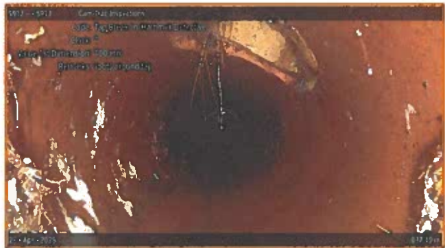
[Grade 3] Tap Break-in/Hammer Defective at 037.40 m, 1 o'clock | roots around tap
