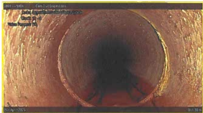
[Grade 2] Deposits Attached Encrustation at 011.30 m, 12 - 4 o'clock
