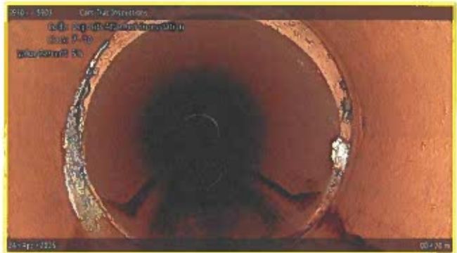
[Grade 2] Deposits Attached Encrustation at 009.20 m, 7 - 10 o'clock
