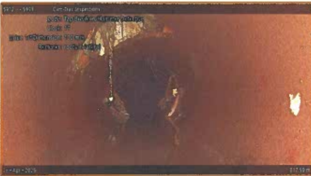
[Grade 3] Tap Break-in/Hammer Defective at 017.50 m, 11 o'clock | roots in lateral
