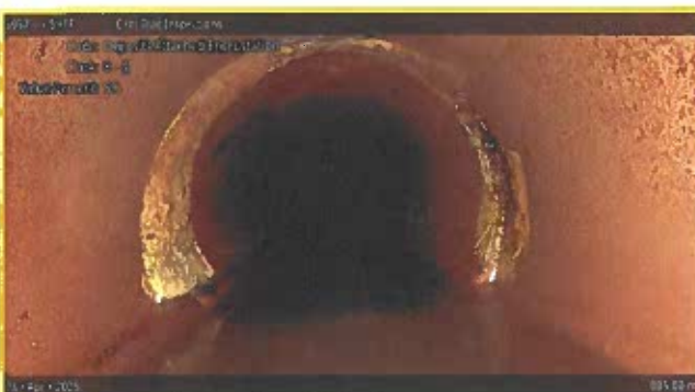
[Grade 2] Deposits Attached Encrustation at 005.00 m, 8 - 4 o'clock
