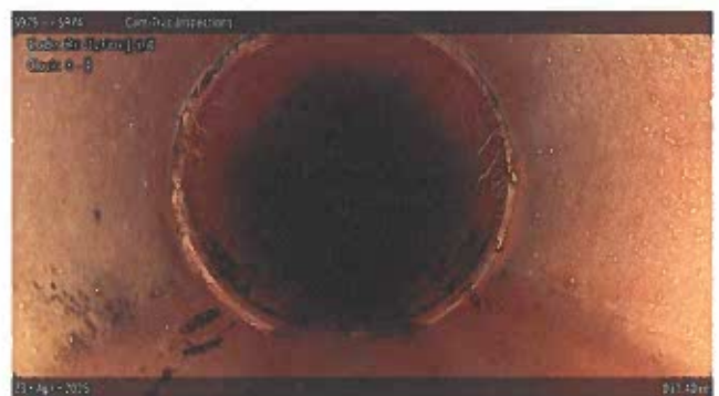
[Grade 1] Roots Fine Joint at 031.40 m, 8 - 4 o'clock
