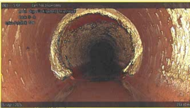
[Grade 2] Deposits Attached Encrustation at 053.40 m, 8 - 4 o'clock
