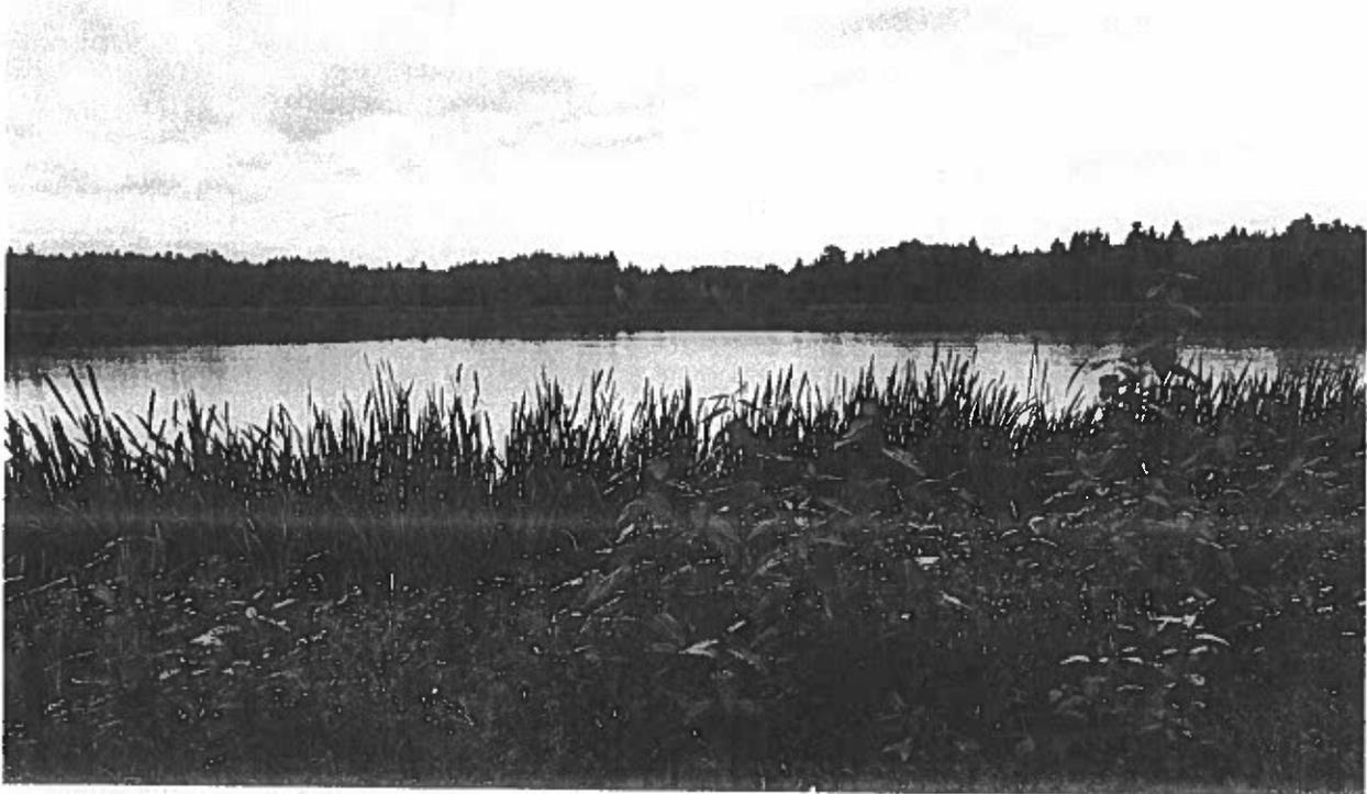
**Figure 6.10: Photo of the Seba Beach Lagoon that is currently closed. The photo depicts the high fluid levels in the lagoon and the overgrowth of vegetation on the berms.**
